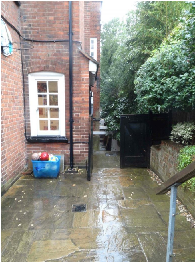
Photograph Three: Rear side elevation (North)
