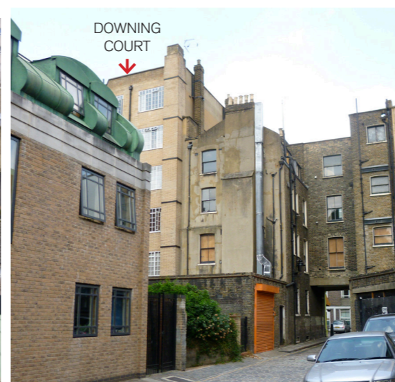
View east along Colonnade
