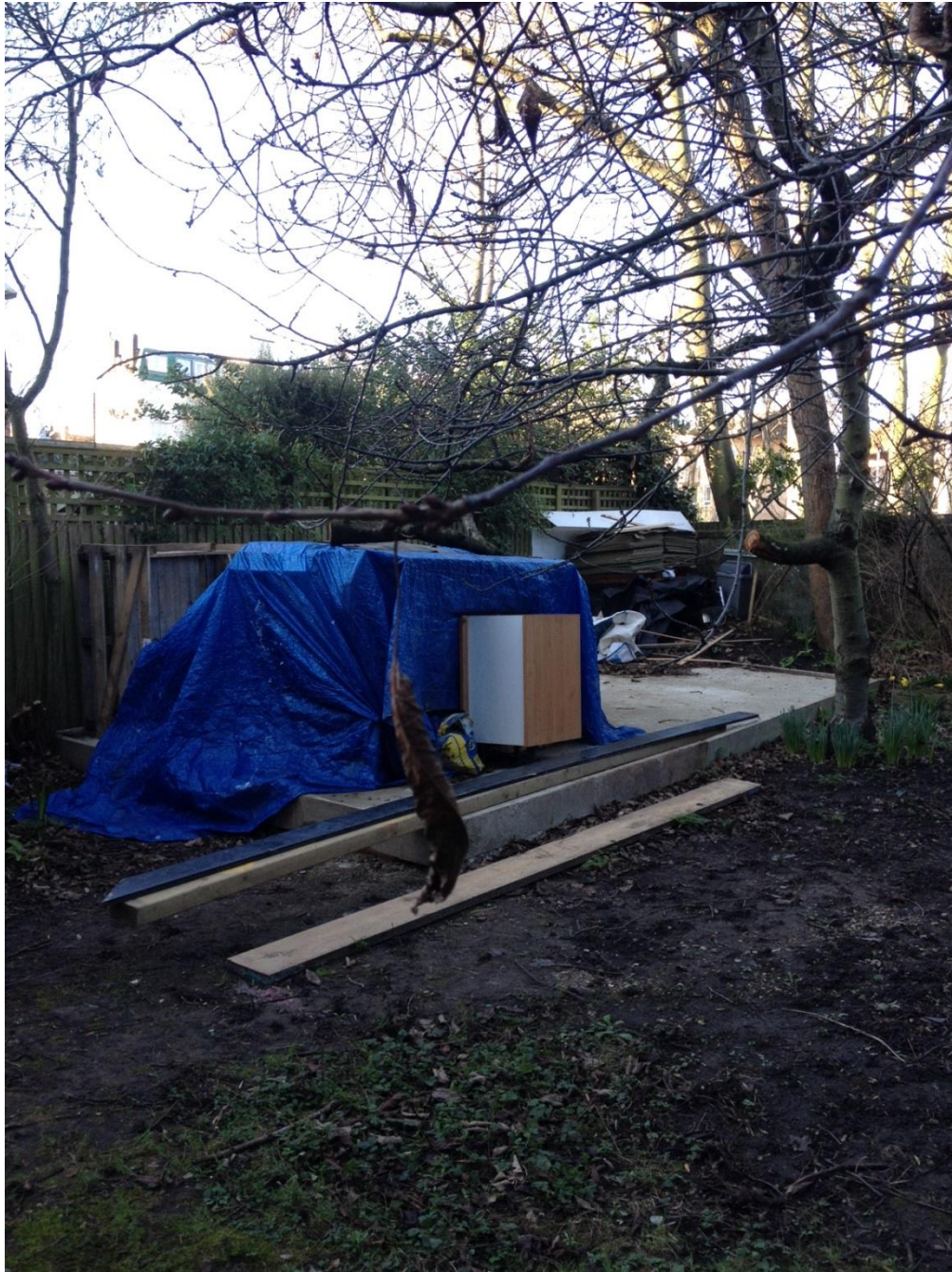
Photo 1- Rear Garden Showing Building Platform
