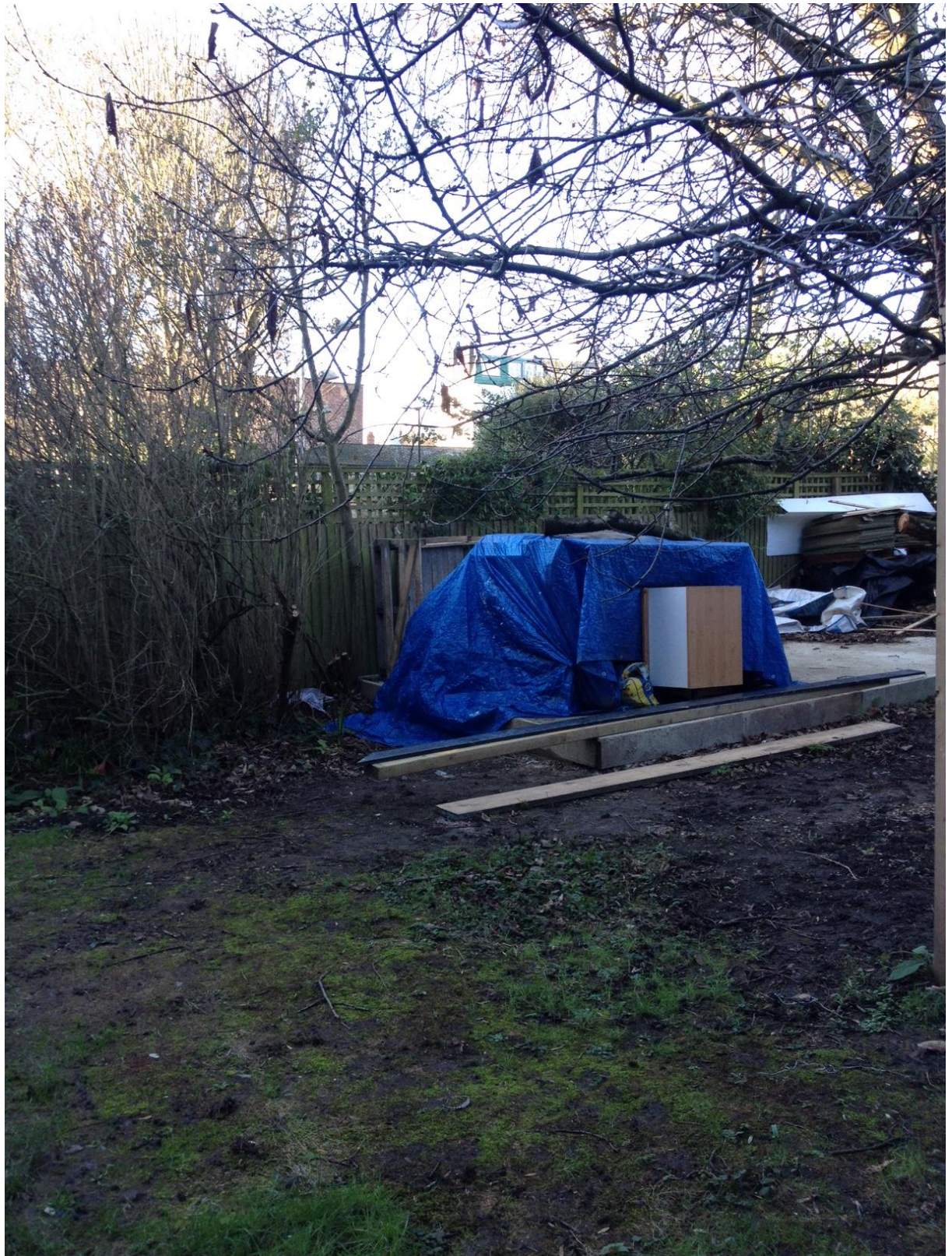
Photo 3- Rear Garden Showing Building Platform
