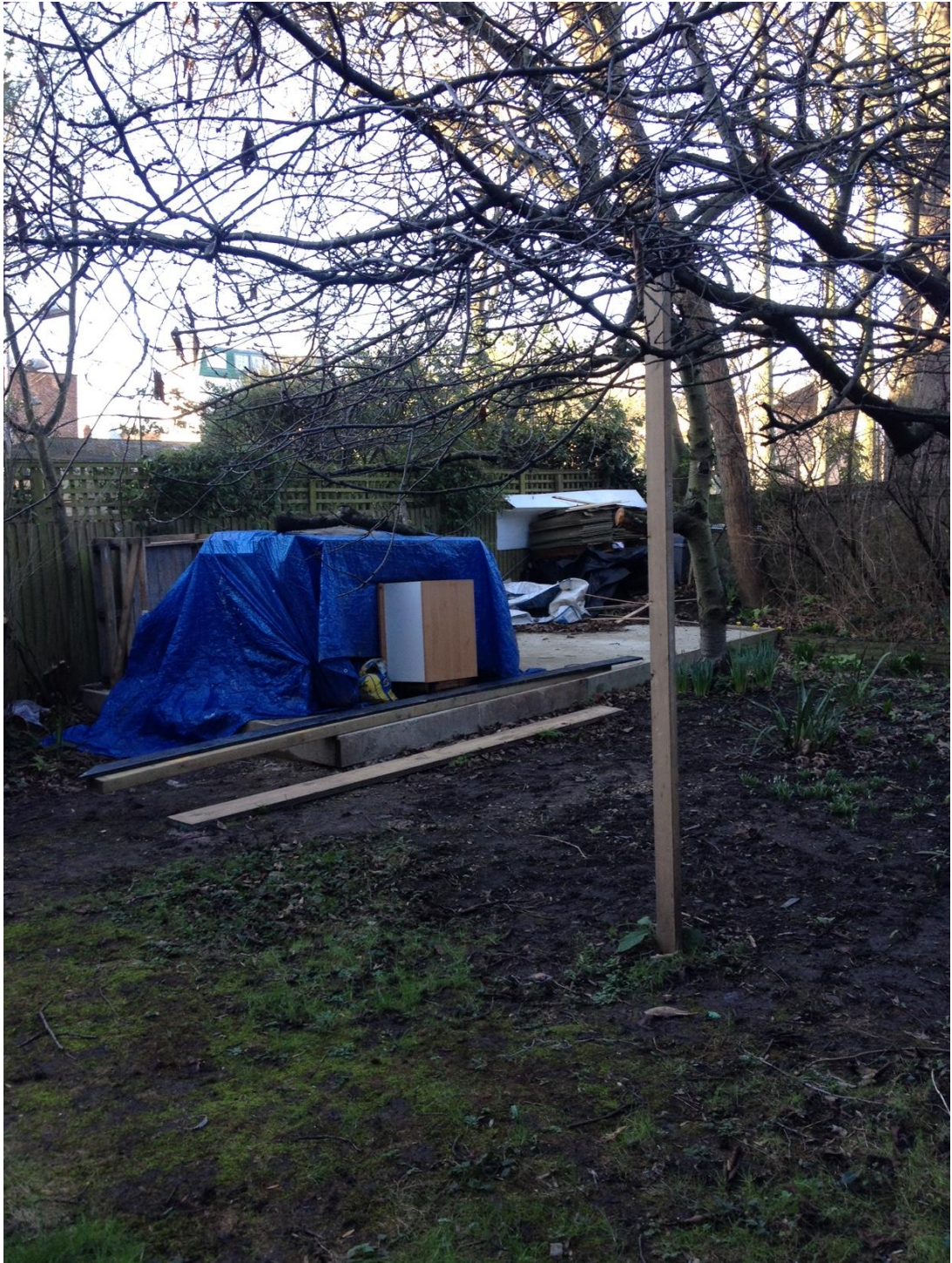
Photo 2- Rear Garden Showing Building Platform
