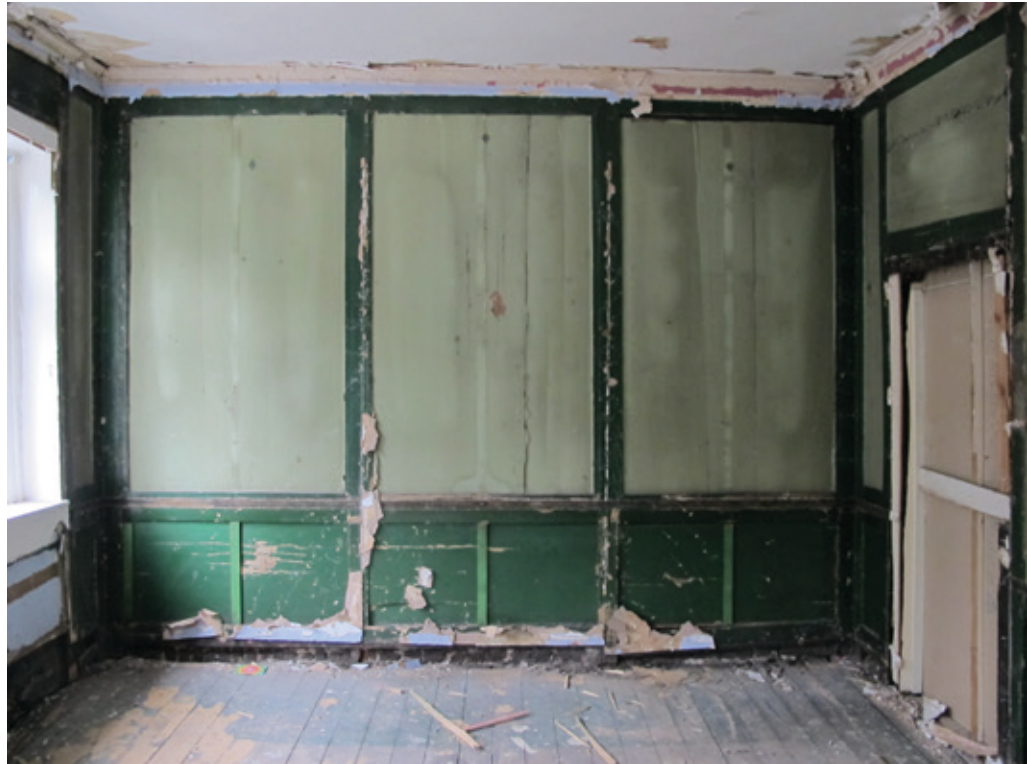
No. 26, second floor front room, showing recently discovered panelling
