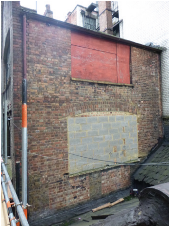
No. 23, north façade, with roof of No. 22 in foreground
