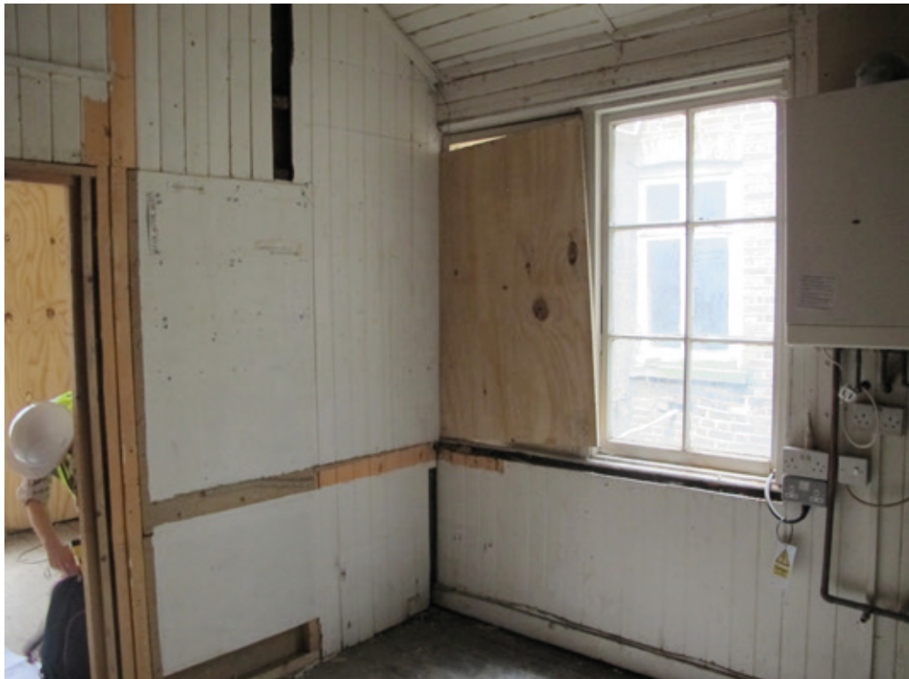
No. 23, second-floor interior
