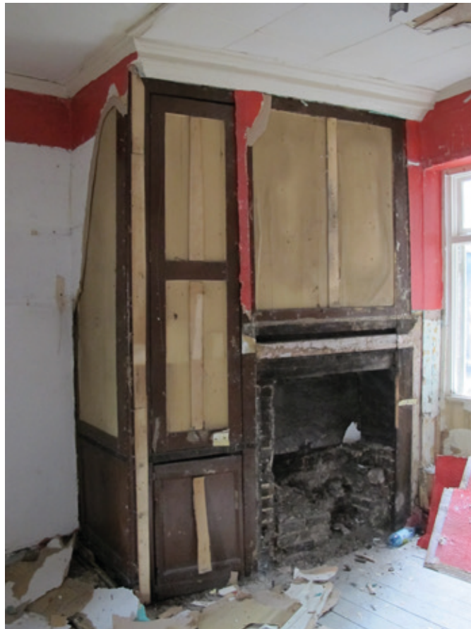
No. 26, second floor rear room, showing the discovery of rare surviving cupboards left of the fireplace (the chimney piece has been removed)
