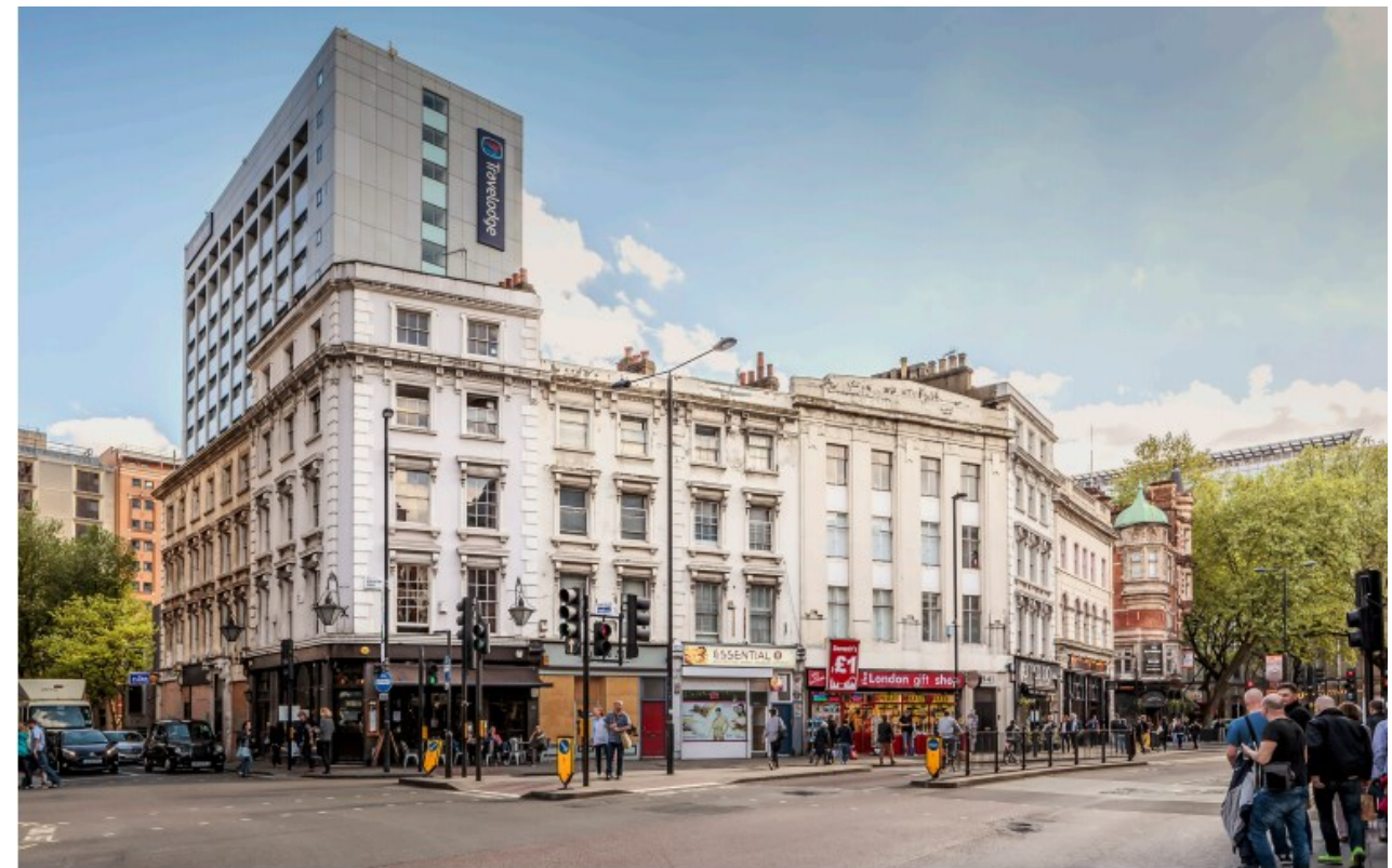
Figure 24. Existing view of nos. 35, 37 and 39-41 New Oxford Street, and 10-12 Museum, Street looking west along New Oxford Street on the corner with High Holborn.
