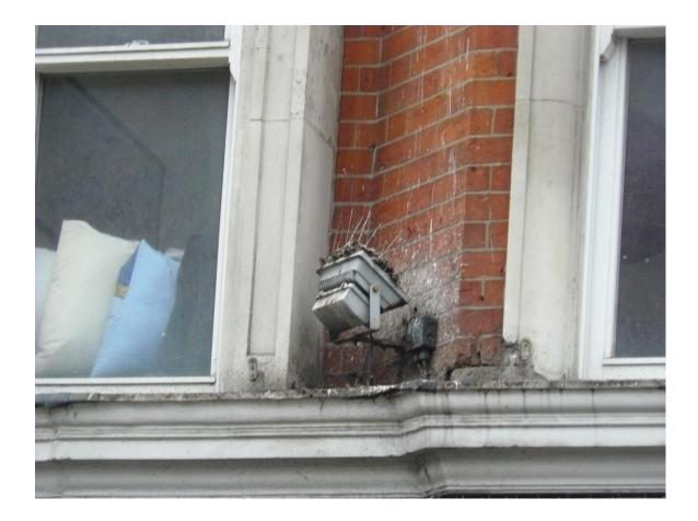
Renew pigeon spikes. Pest control measures are all damaged or defective, renew spikes throughout elevation.
