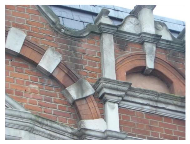
Check coping stone secure. Clean down all loose and soluble soot and dirt deposits from the elevation using fine nebulous sprays of clean cold water controlled with an intermittent pulse spray. Rinse down thoroughly using low pressure Doff steam cleaning process.
