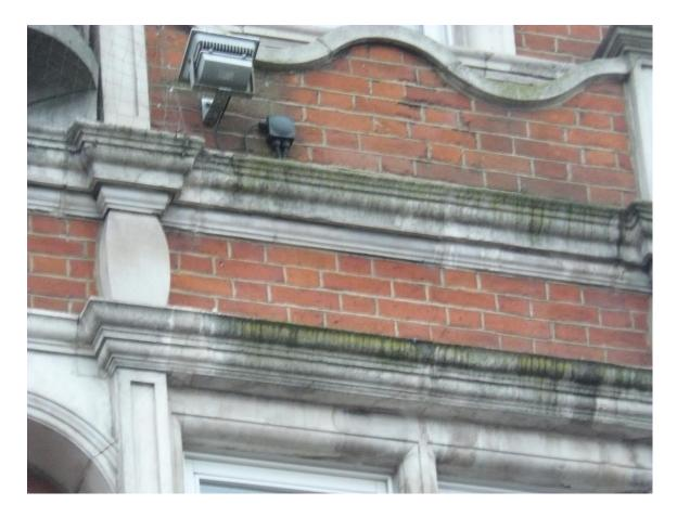
Commencing from roof level to 1st floor, thoroughly clean down all loose and soluble soot and dirt deposits from the elevation using fine nebulous sprays of clean cold water controlled with an intermittent pulse spray. Rinse down thoroughly using low pressure Doff steam cleaning process to cornices.
