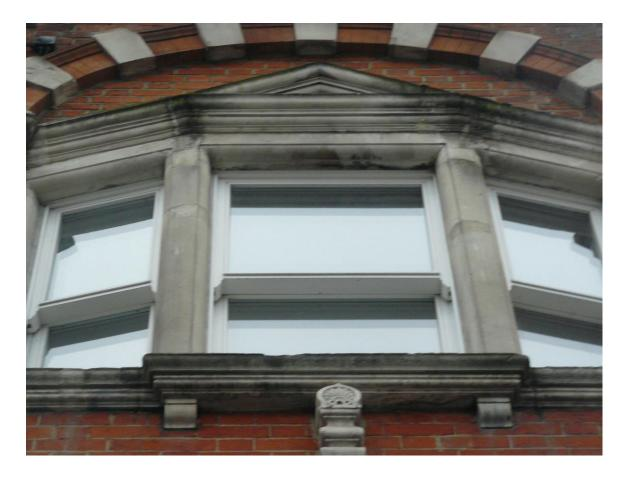
Inspect damage to window sills, remove all accumulated dirt. Make good like for like any damage to sills in situ.
