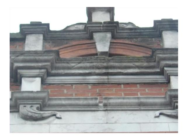
Inspect damage to cornices, remove all accumulated dirt. Make good like for like any damage to cornice in situ.
