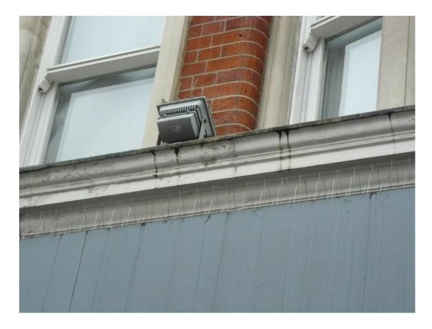
Inspect damage to lintels, remove all accumulated dirt. Make good like for like any damage to lintels in situ.
