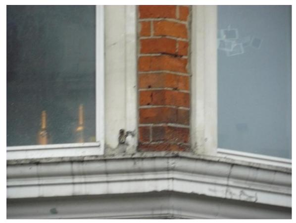
To areas of defective brick pointing, carefully cut out using suitable diamond blade/suitable quirks and chisels to a depth of at least 10mm or twice the joint width. Dust out, damp and re-point in lime based gauged mortar to match existing in every respect. Carefully wash off residues from adjacent areas.
