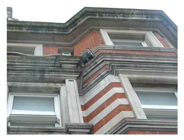
Commencing from roof level to 1st floor, thoroughly clean down all loose and soluble soot and dirt deposits from the elevation using fine nebulous sprays of clean cold water controlled with an intermittent pulse spray. Rinse down thoroughly using low pressure Doff steam cleaning process to stonework.
