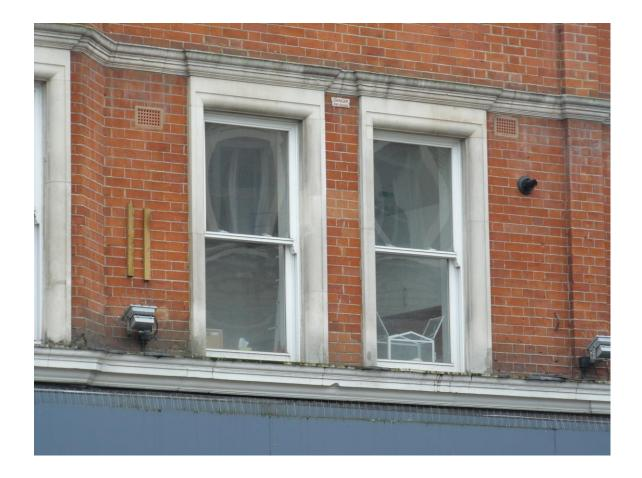
Inspect damage to lintels, remove all accumulated dirt. Make good like for like any damage to lintels in situ.
