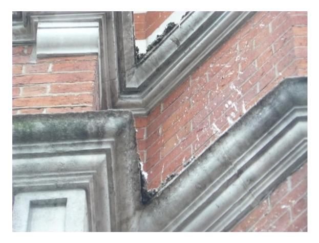
Commencing from roof level to 1st floor, thoroughly clean down all loose and soluble soot and dirt deposits from the elevation using fine nebulous sprays of clean cold water controlled with an intermittent pulse spray. Rinse down thoroughly using low pressure Doff steam cleaning process to brickwork.
