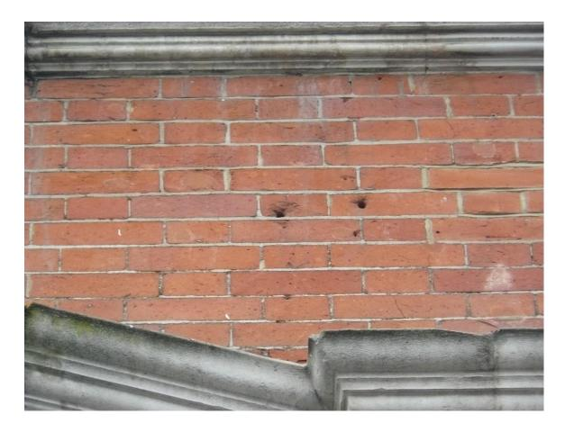
To areas of defective brick pointing, carefully cut out using suitable diamond blade/suitable quirks and chisels to a depth of at least 10mm or twice the joint width.
