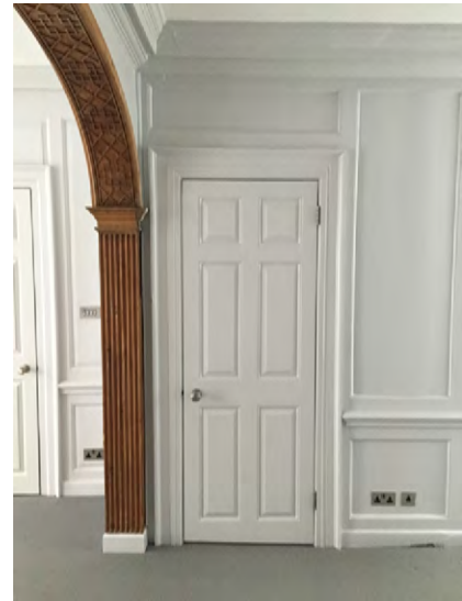
Fig. 33- Ground Floor Timber Detailing
