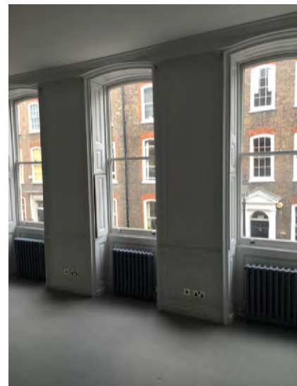
Fig. 36 - First Floor Front Facade
