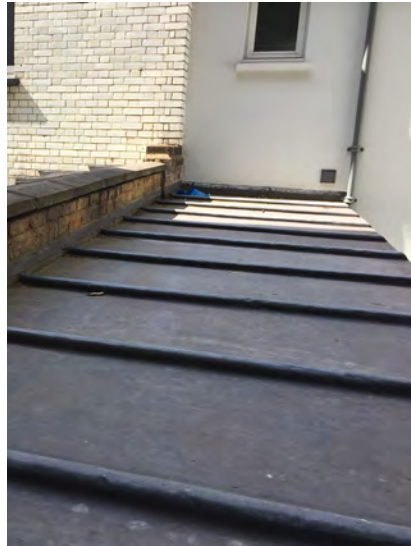
Fig. 16 - Link Roof to Annex
