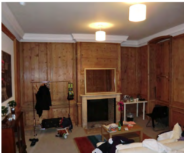
Fig. 07 - Exposed Panelling at First Floor
