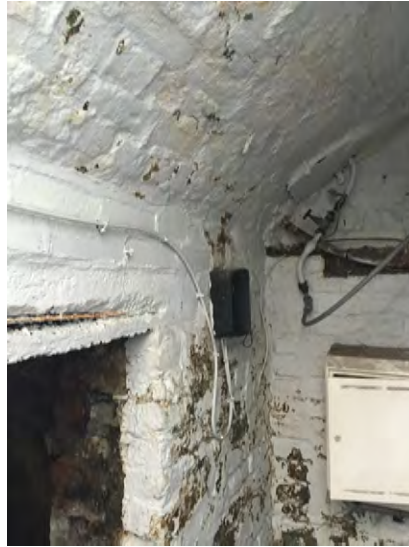
Fig. 26 - Lower Ground Front Entrance Services
