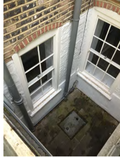
Fig. 14 - Light-well to Basement level
