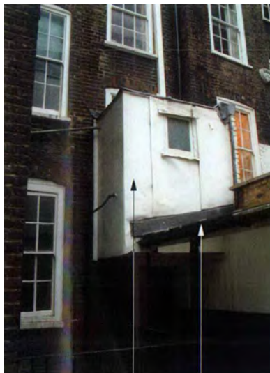
Fig. 06 - Previous Toilet Pod
