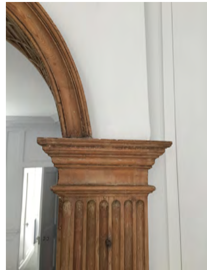
Fig. 24 - Ground Floor Timber Detailing
