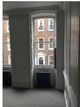
Figure 11 – Cornice and Shutters (first floor)
