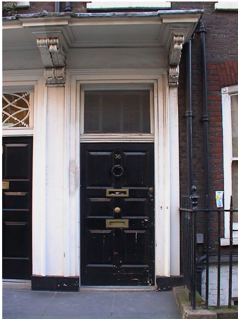
Figure 7 – Existing Entrance Doorway Showing Plain Fanlight
