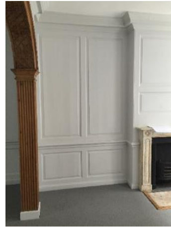
Figure 9 – Existing Panelling (ground floor)
