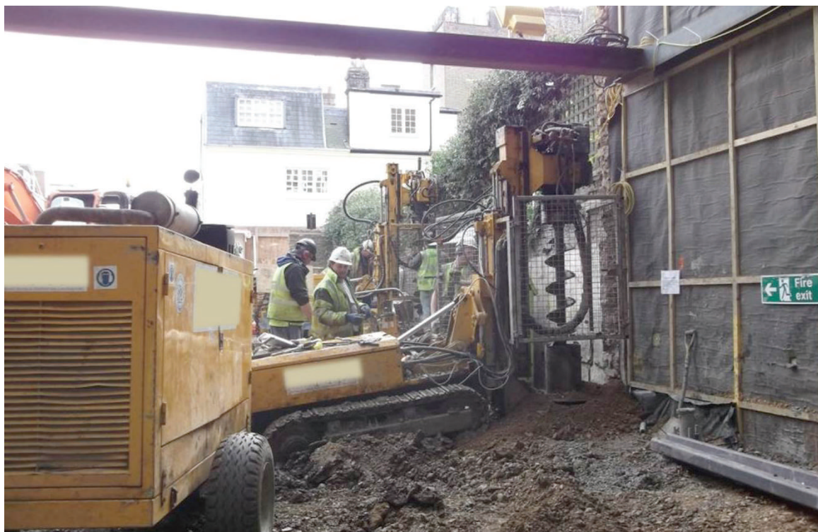
Figure 4 Piling rig at work within basement
