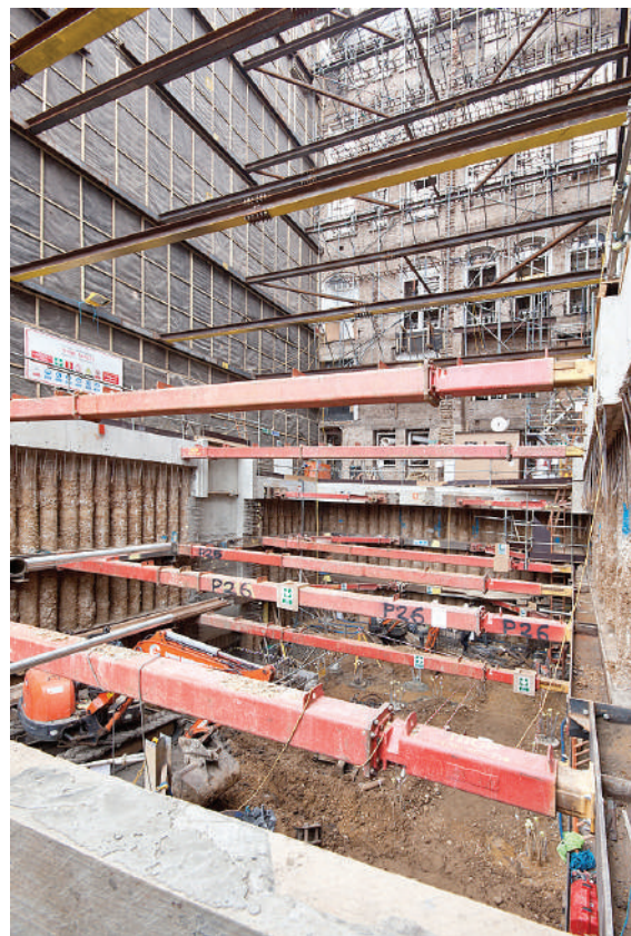
Figure 3 Propping scheme (1st level) looking towards Pont Street
