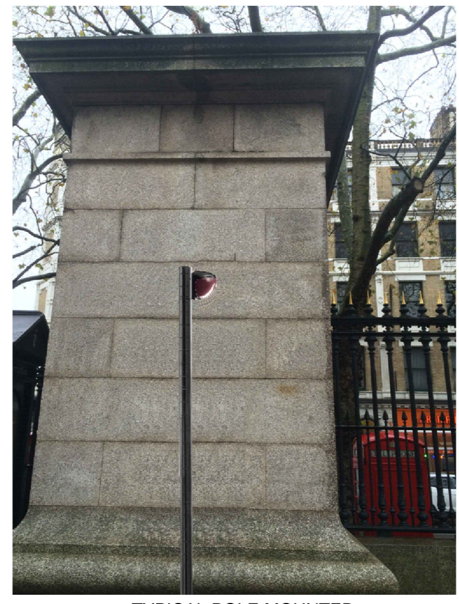
TYPICAL POLE MOUNTED PIR DETECTOR EXAMPLE
