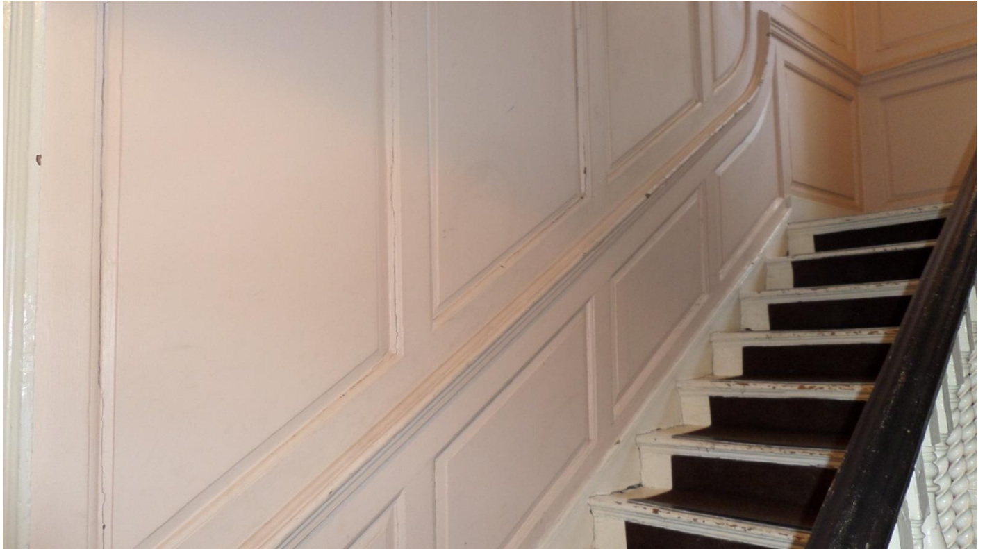
Fig3 Panelling to the Stairs
