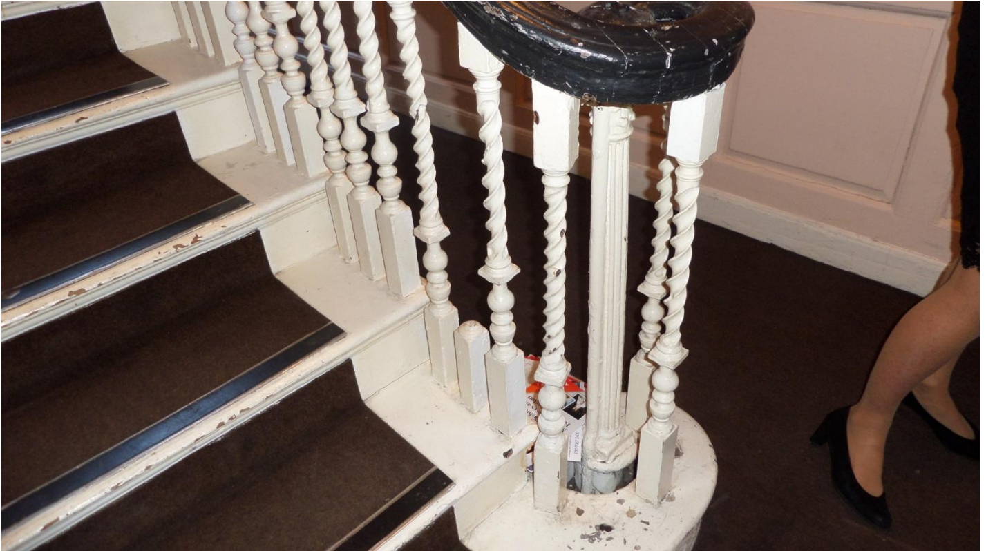
Fig 8 Areas highlighting missing balusters
