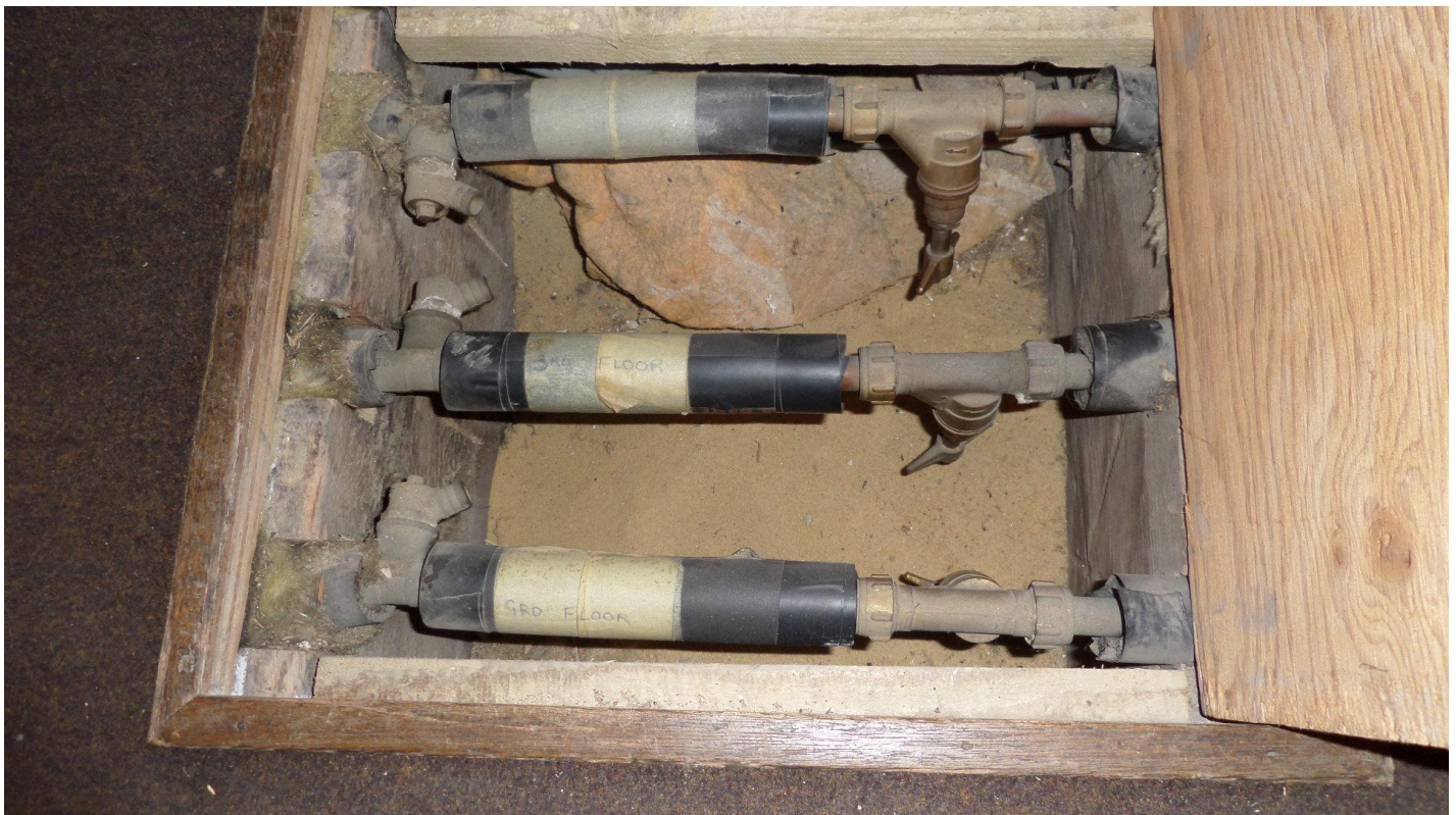
Fig 11 Original sand pugging
