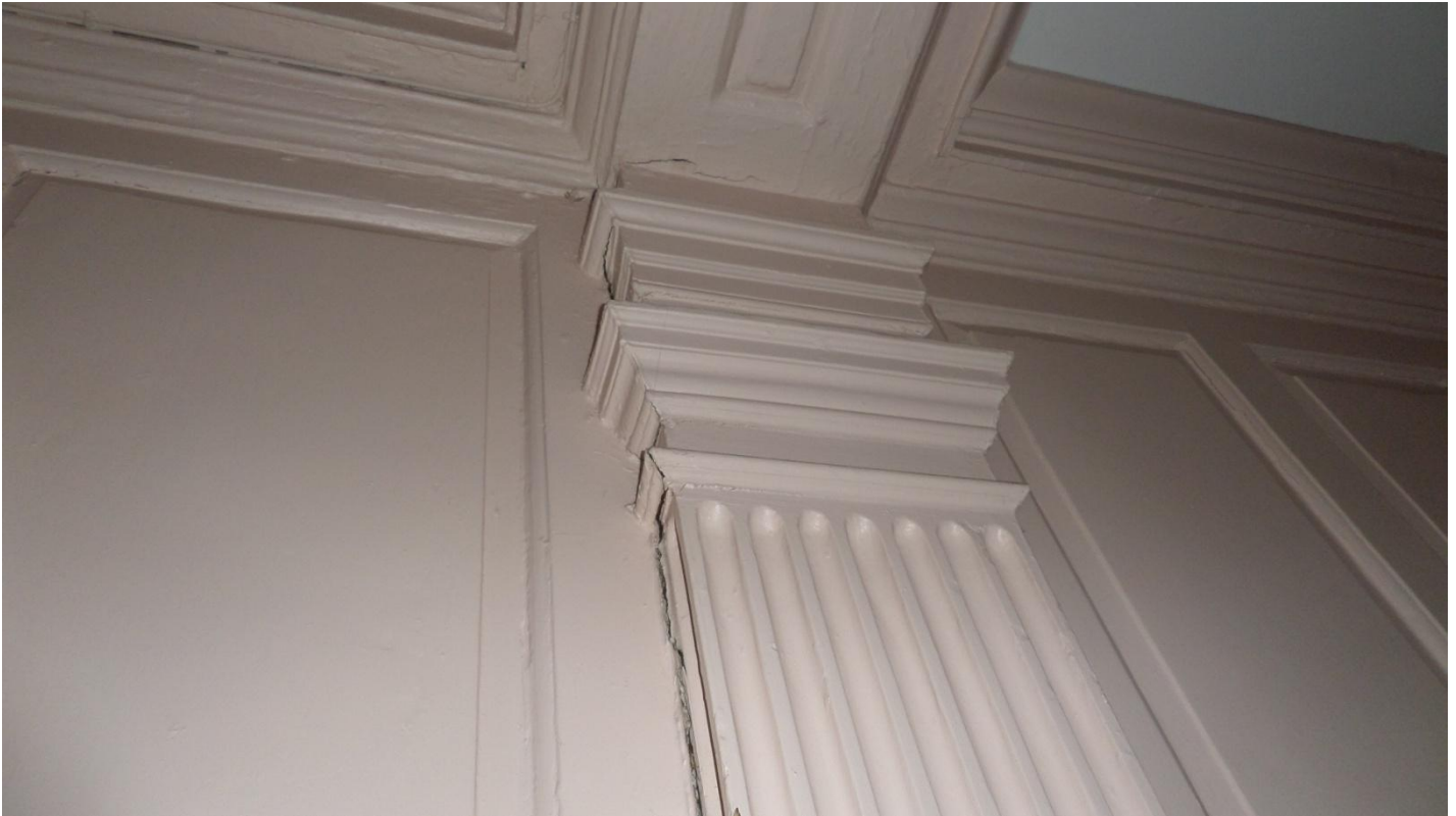
Fig6 Splits associated with thermal movement or drying out of the timber
