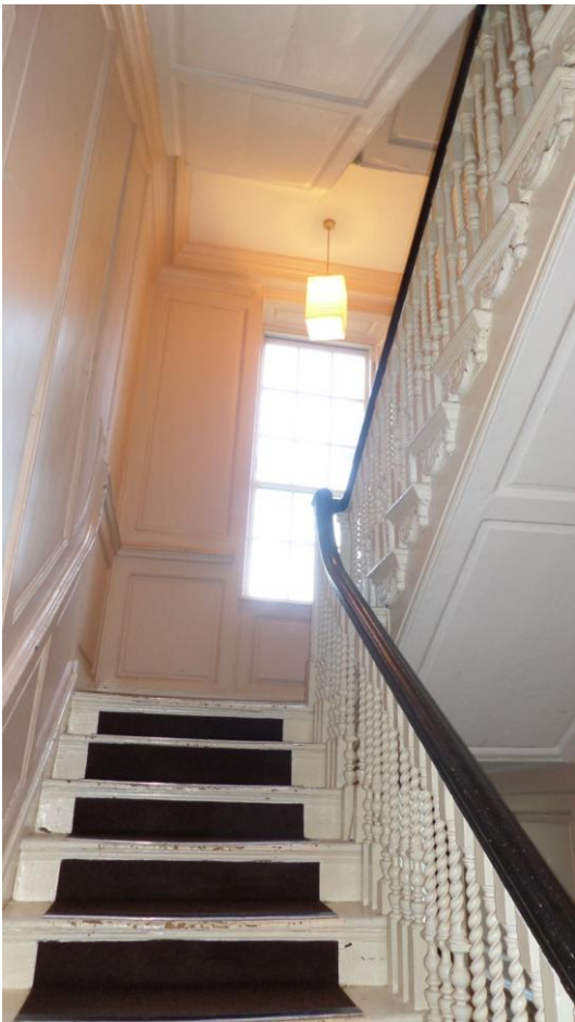
Fig 9 Decorative tread ends to the staircase
