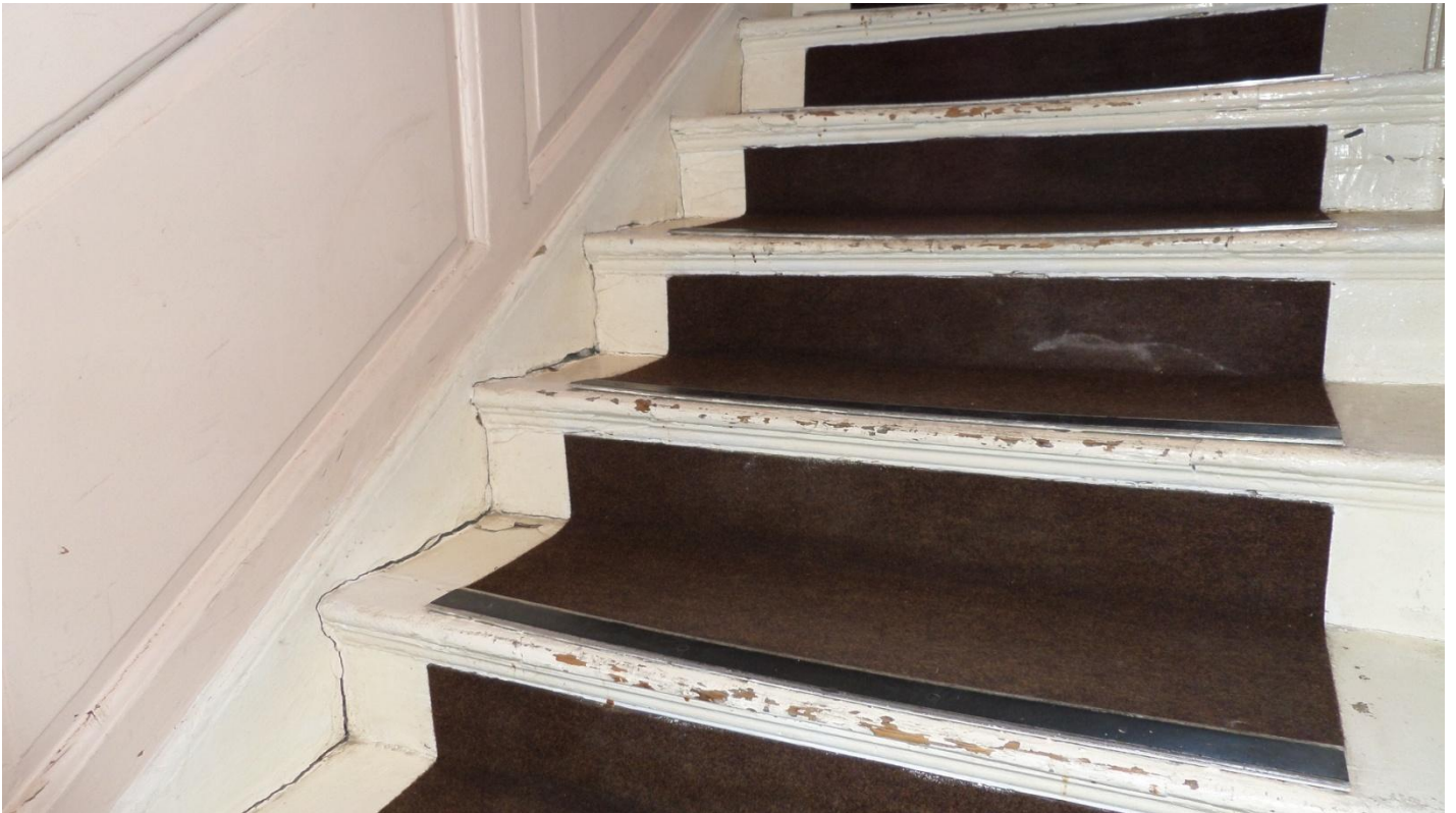
Cracks highlighting the failing end bearers
