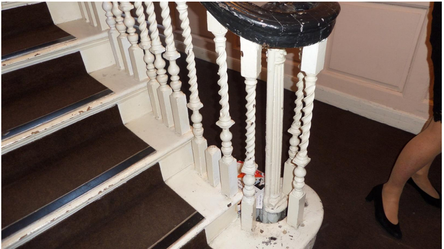
Stair case, evidence of missing balusters
