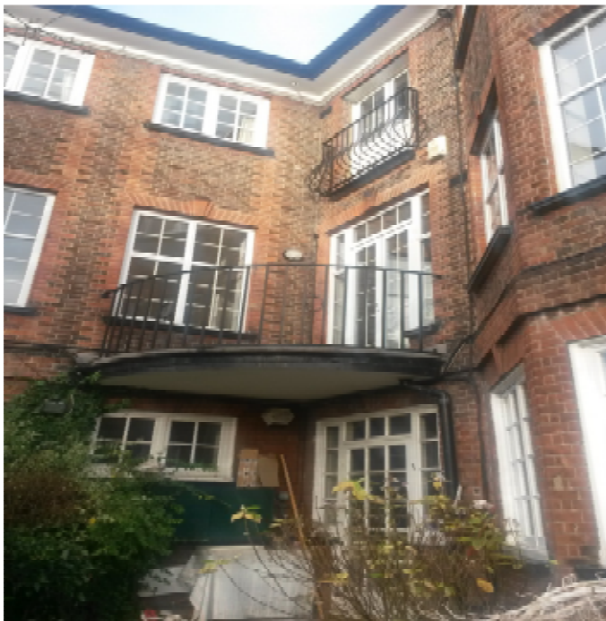
2. Conservatory location with neighbouring flats above.
