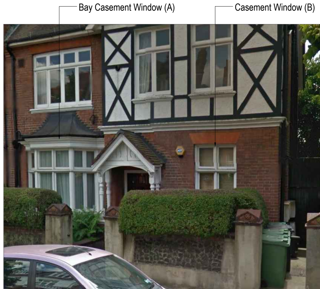
Existing Ground Floor Windows Bay Casement Window and adjacent Casement Window
