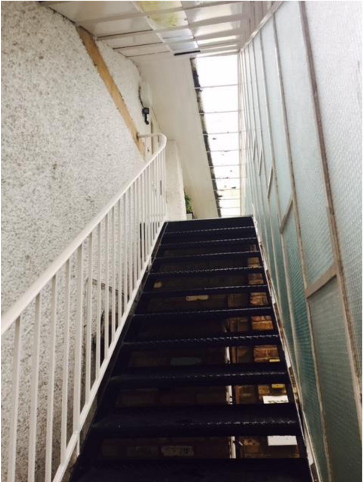
View looking down the external stair case
