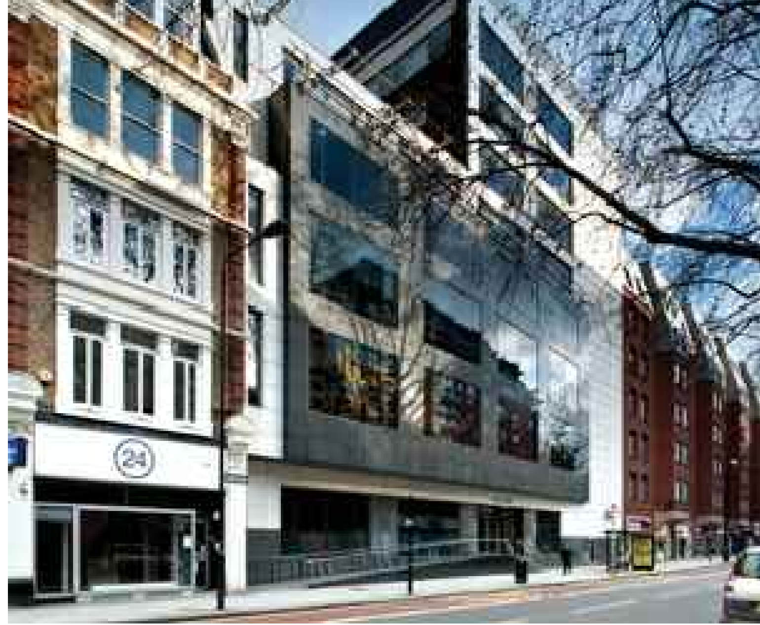
EXISTING PHOTO FOX COURT FRONT FACADE, GRAYS INN ROAD
