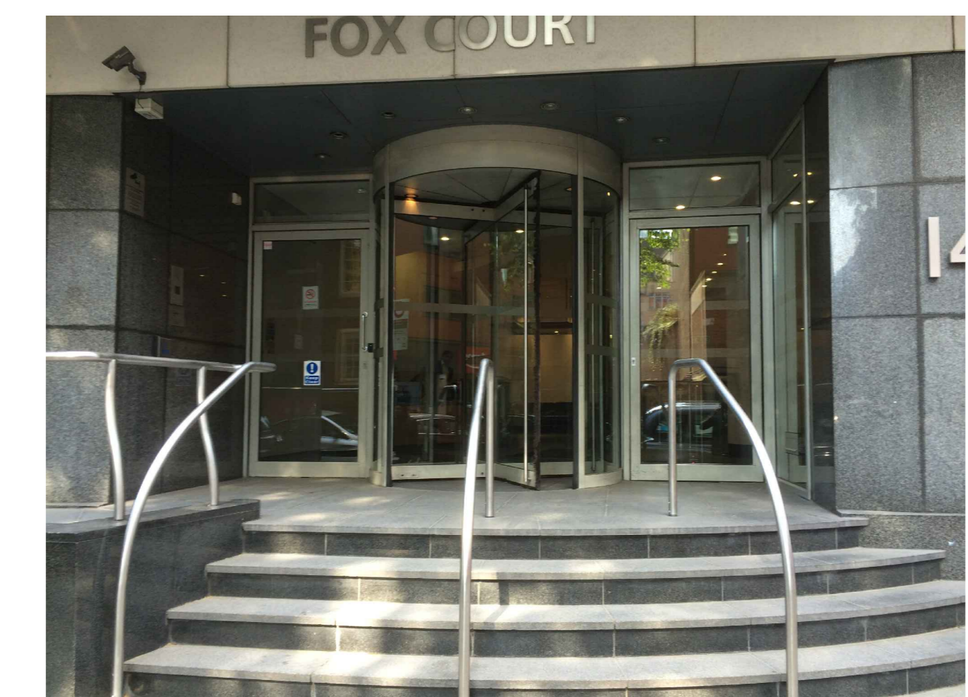
EXISTING PHOTOS FOX COURT ENTRANCE, GRAYS INN ROAD
