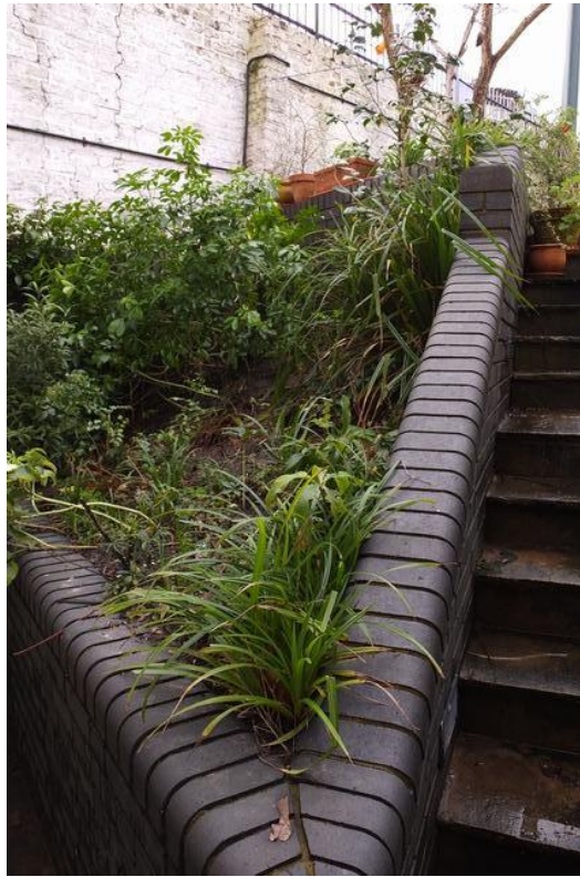
Image 7 Showing the significant drop between the raised beds
