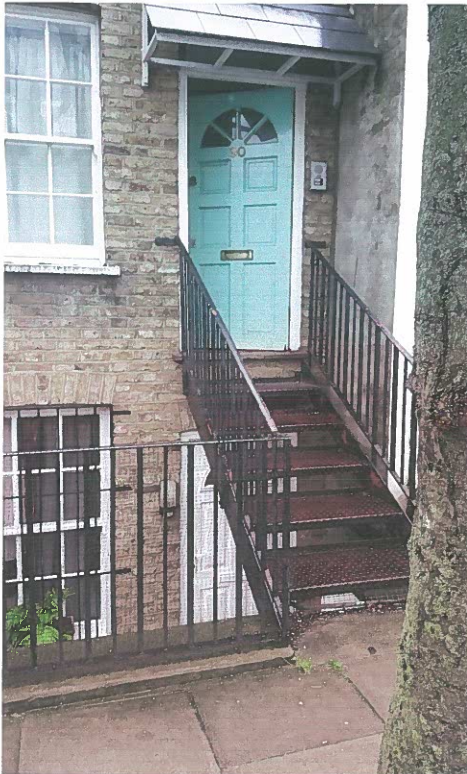
Photo 1: Stairs to main entrance to existing flat
