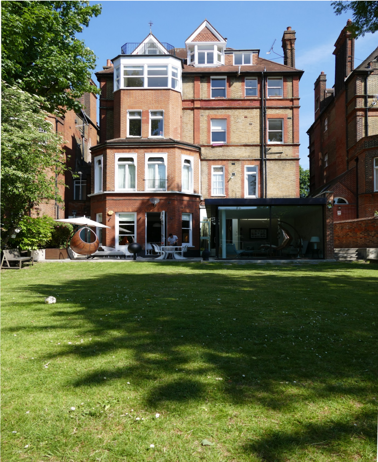
Existing Rear Extension
