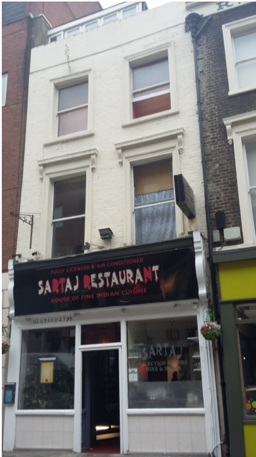
Front of building
