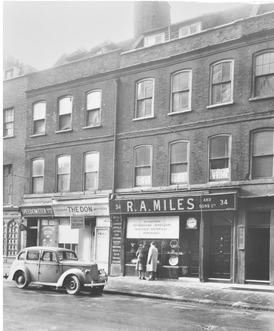
Figure 8: Photograph dating to 1945, showing the ground floor of 35 Great Queen Street subdivided into two units. It also shows earlier windows than the current windows, although these are not original
