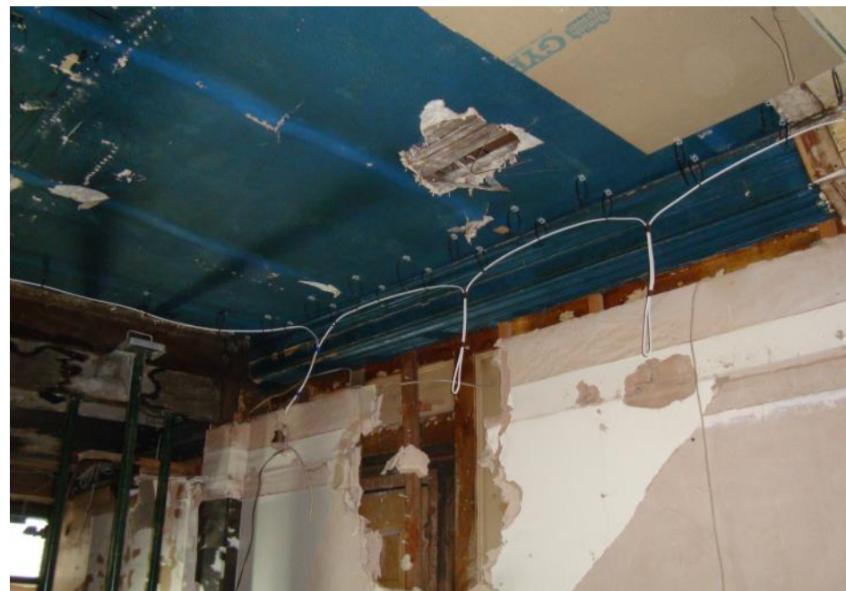
Figure 22: Cornicing and historic ceiling survive above the suspended ceiling, although the condition is poor in places.
