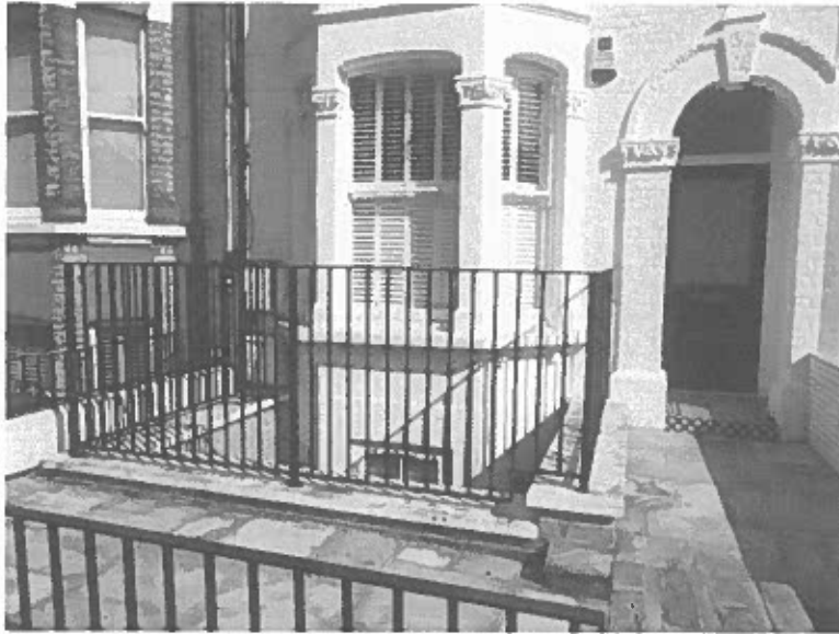
Photo 6 – Lightwell to front of building with mild steel handrails around well.
