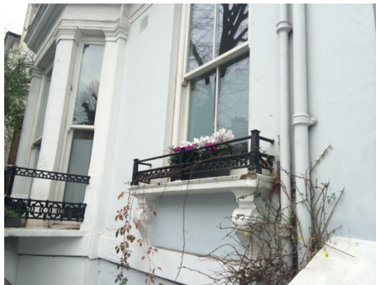
PHOTOGRAPH 13 : Existing Wrought Iron Detailing
