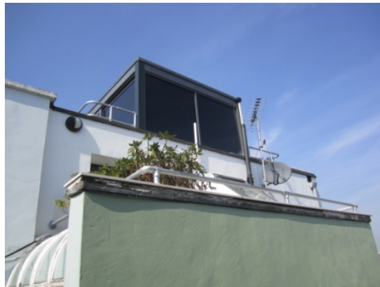
PHOTOGRAPH 12 : View of existing roof extension from No. 36 Regents Pk Rd
