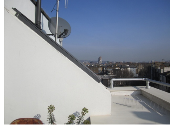
PHOTOGRAPH 10 : Third Floor Extension – over stair
