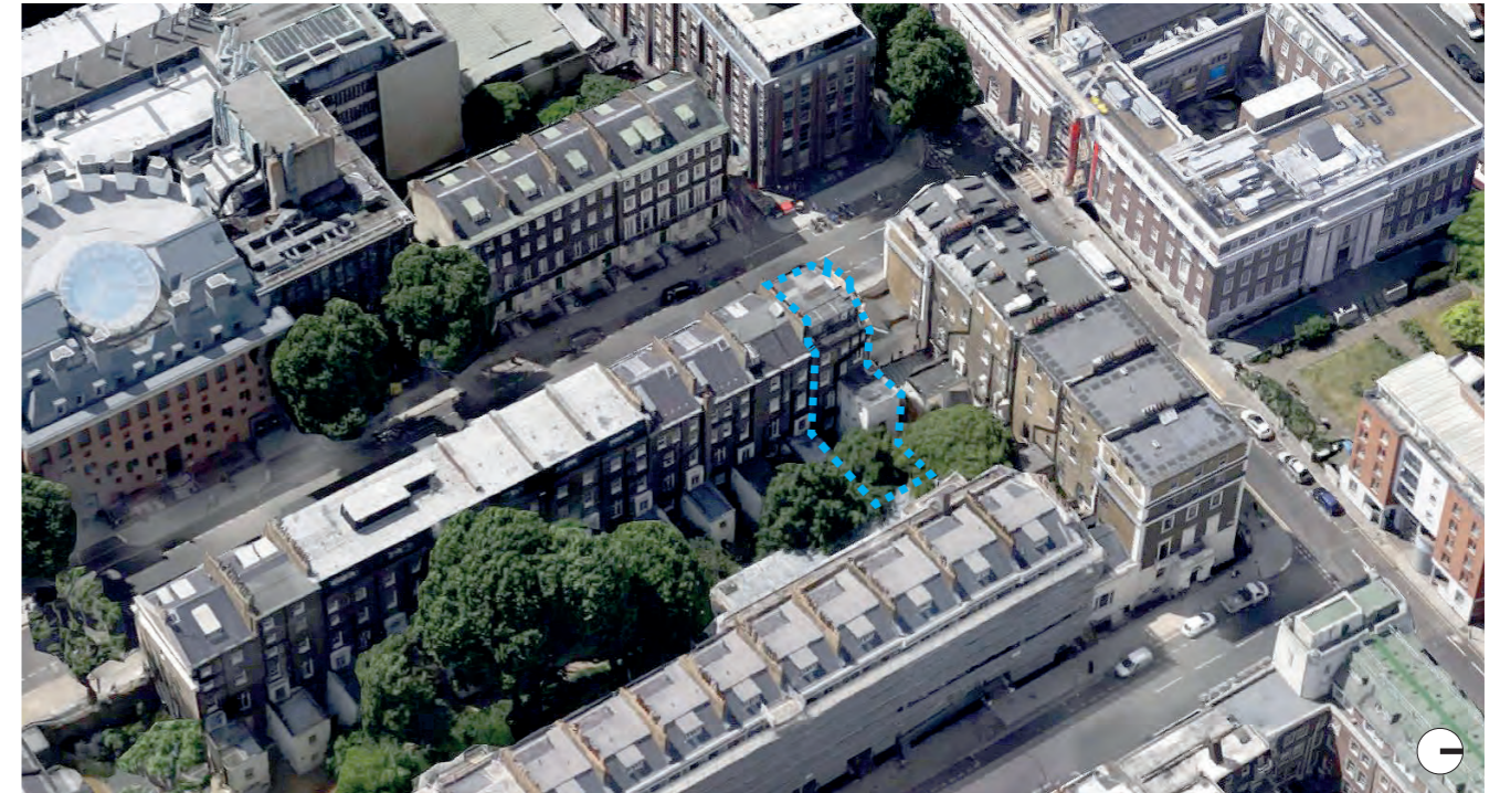
▲ Aerial View of site from east
