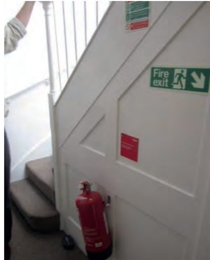
View 2 : Third floor landing and base of stairs
