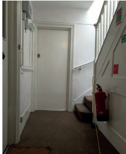
View 1 : Third floor landing
