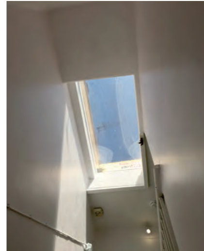
View 4 : Stairs to fourth floor, looking up
