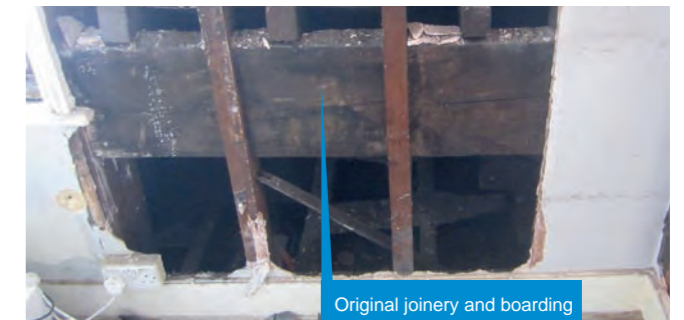
Lining opened up, showing roof framing (old timber) and hardwood studs
