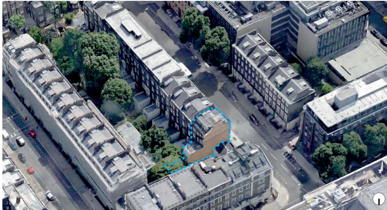
▲ Aerial View of site from north
