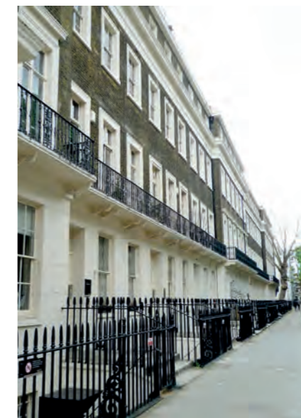
▲ View of pavement level railings and first floor balcony
