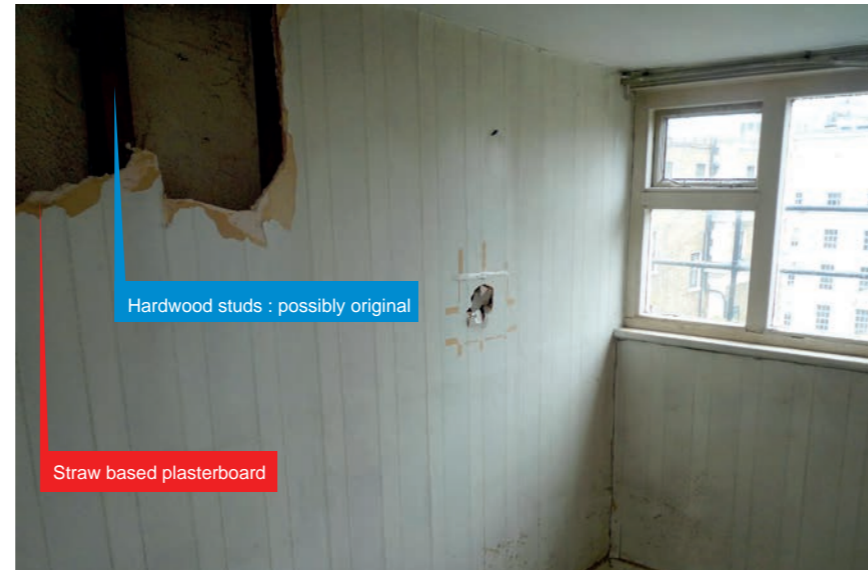
Partition between bedroom 2 and kitchen, view from bedroom.
