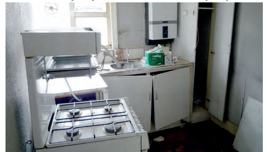
View 7 : Existing east facing kitchen
