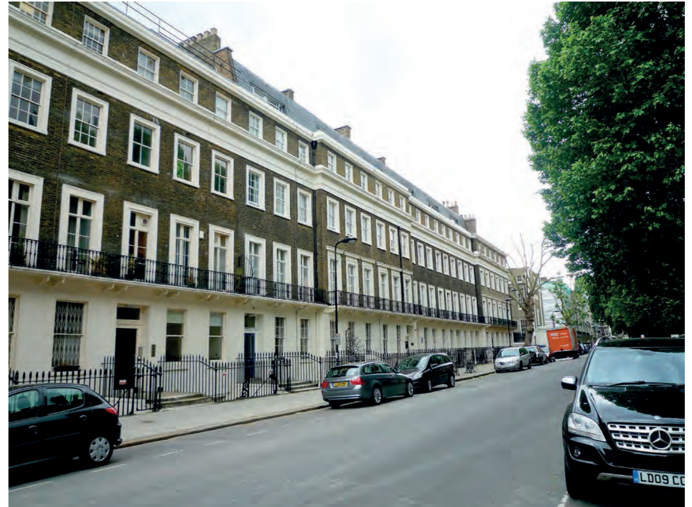
▲ View of Grade II Listed terrace, looking south down Taviton Street
