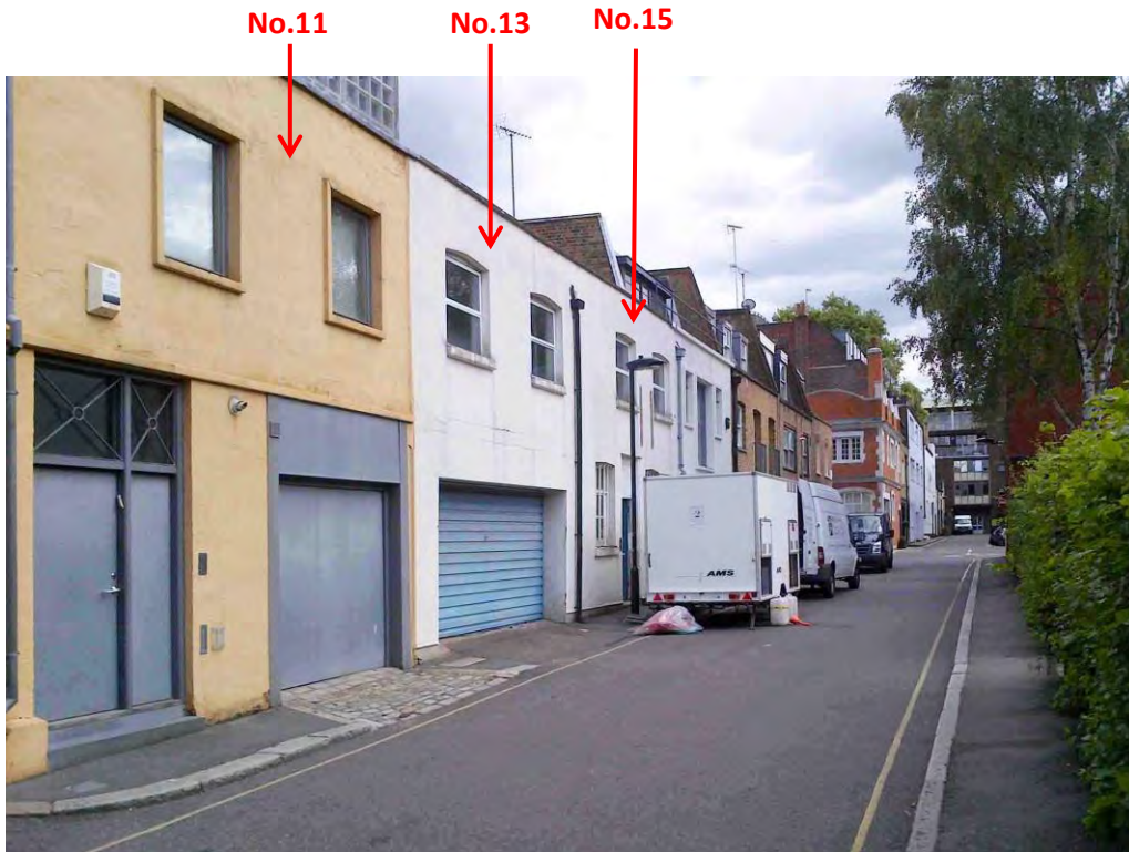
Photo 1: Front elevations of terrace looking south (uphill)
