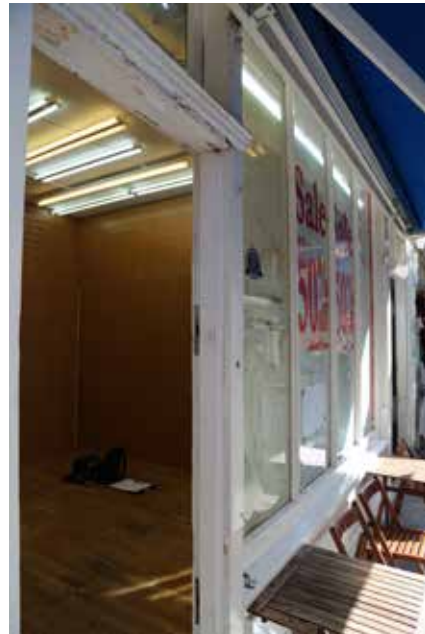
38 Museum Street existing shopfront
