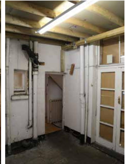
38 Museum Street existing rear yard
