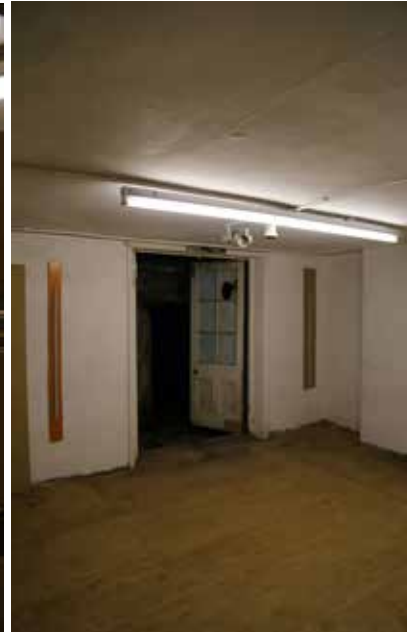
Existing lower ground front room
