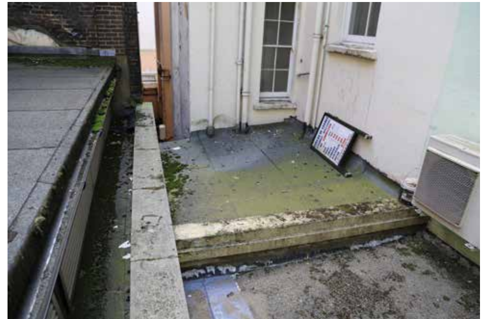
38 Museum Street existing rear canopy, viewed from above on parapet wall
