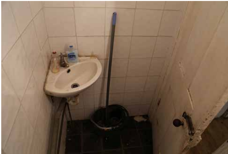
38 Museum Street existing rear WC
