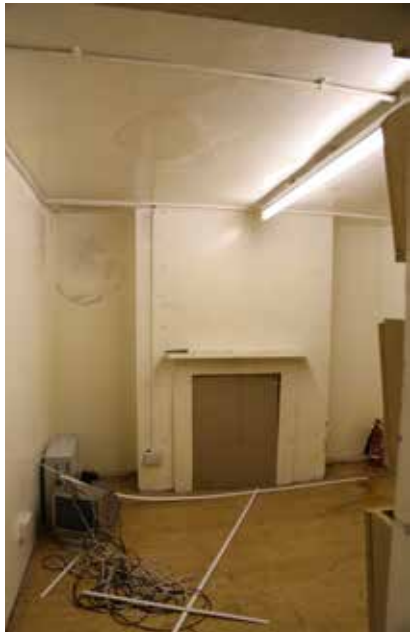
Existing lower ground rear room
