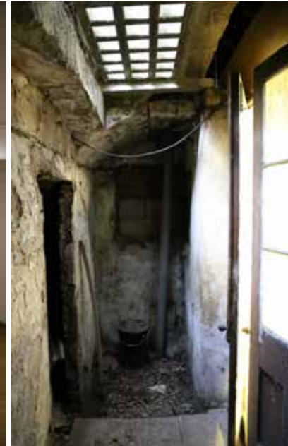
Existing lower ground vaults
