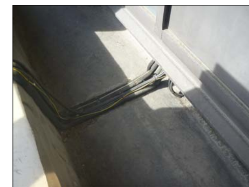
Survey photos of proposed location
