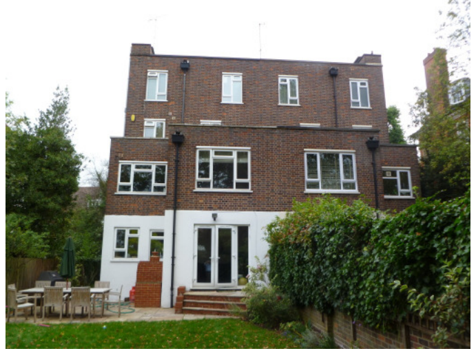
View from the rear showing no.19 obscured at garden level
