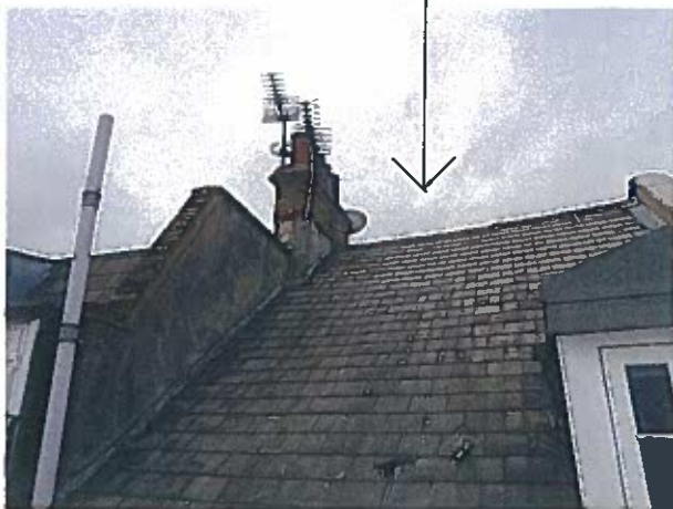
view of rear roof of no.48
