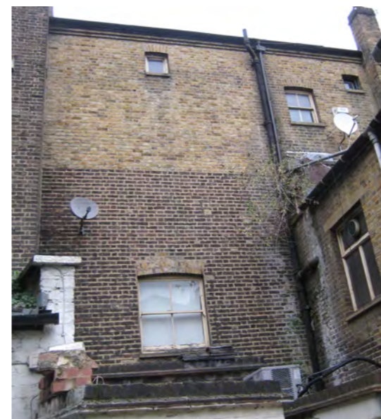
Photo. 5 Existing main rear wall elevation.
