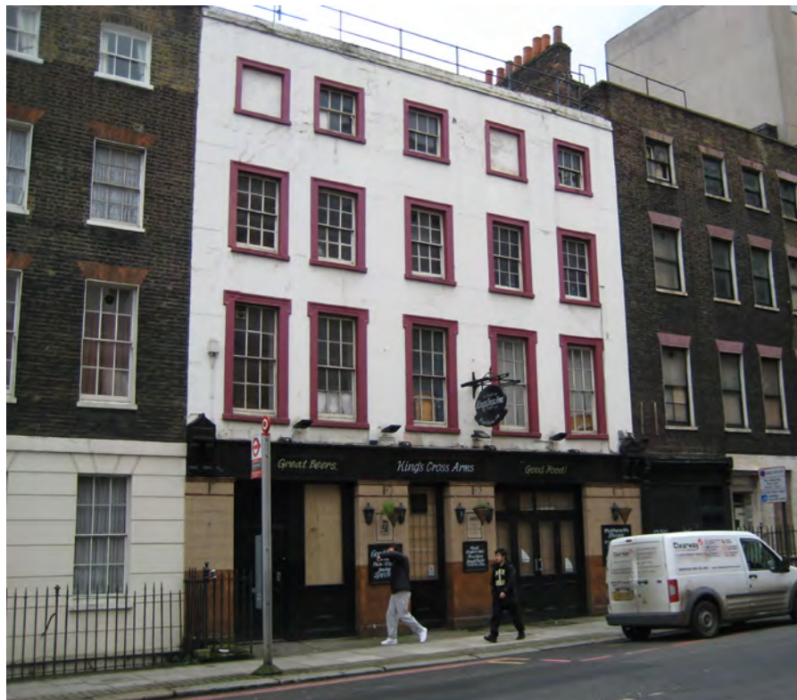
Photo. 7 Existing front elevation
