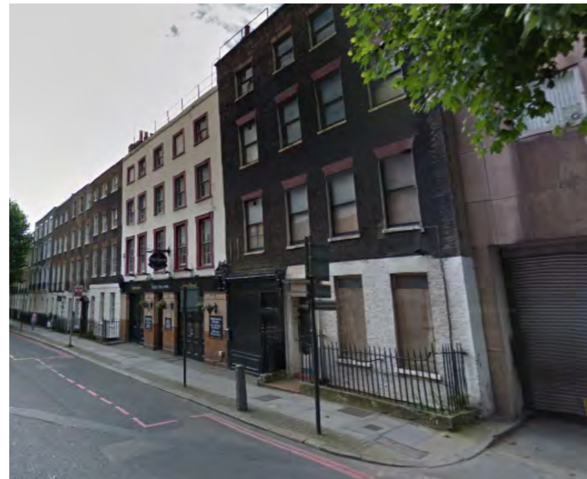
Photo. 1 Existing front elevation from Swinton Street looking East
