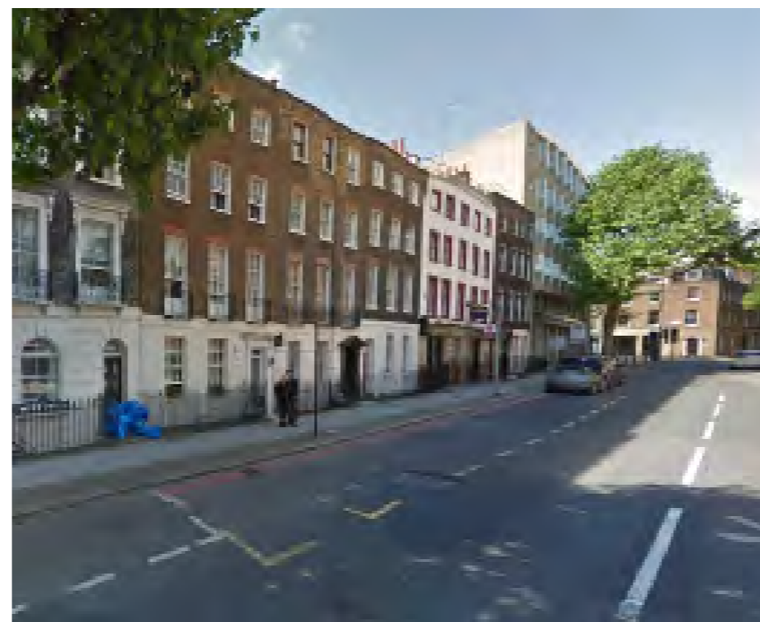
Photo. 3 Existing front elevation from Swinton Street looking West
