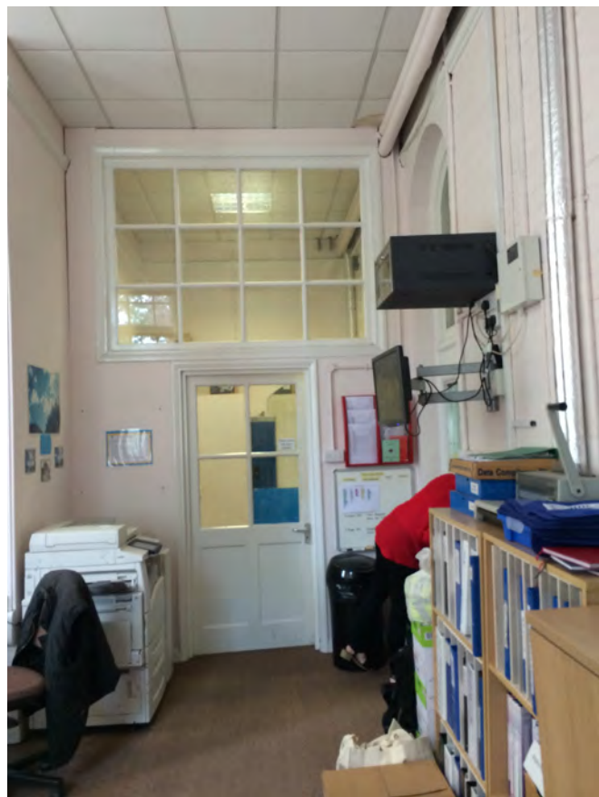
2 Go2 Main office facing south
