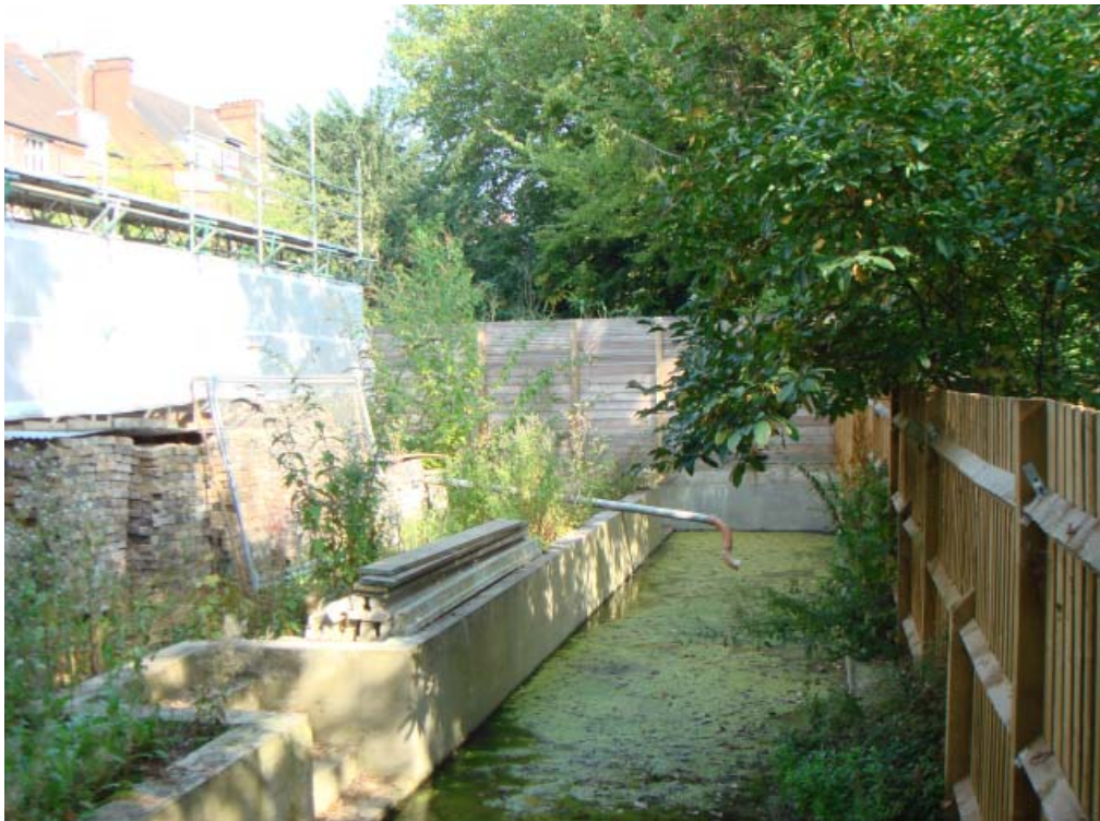
Existing concrete sub-surface 'box' to be infilled and converted into SUDS system with grassed surface.
