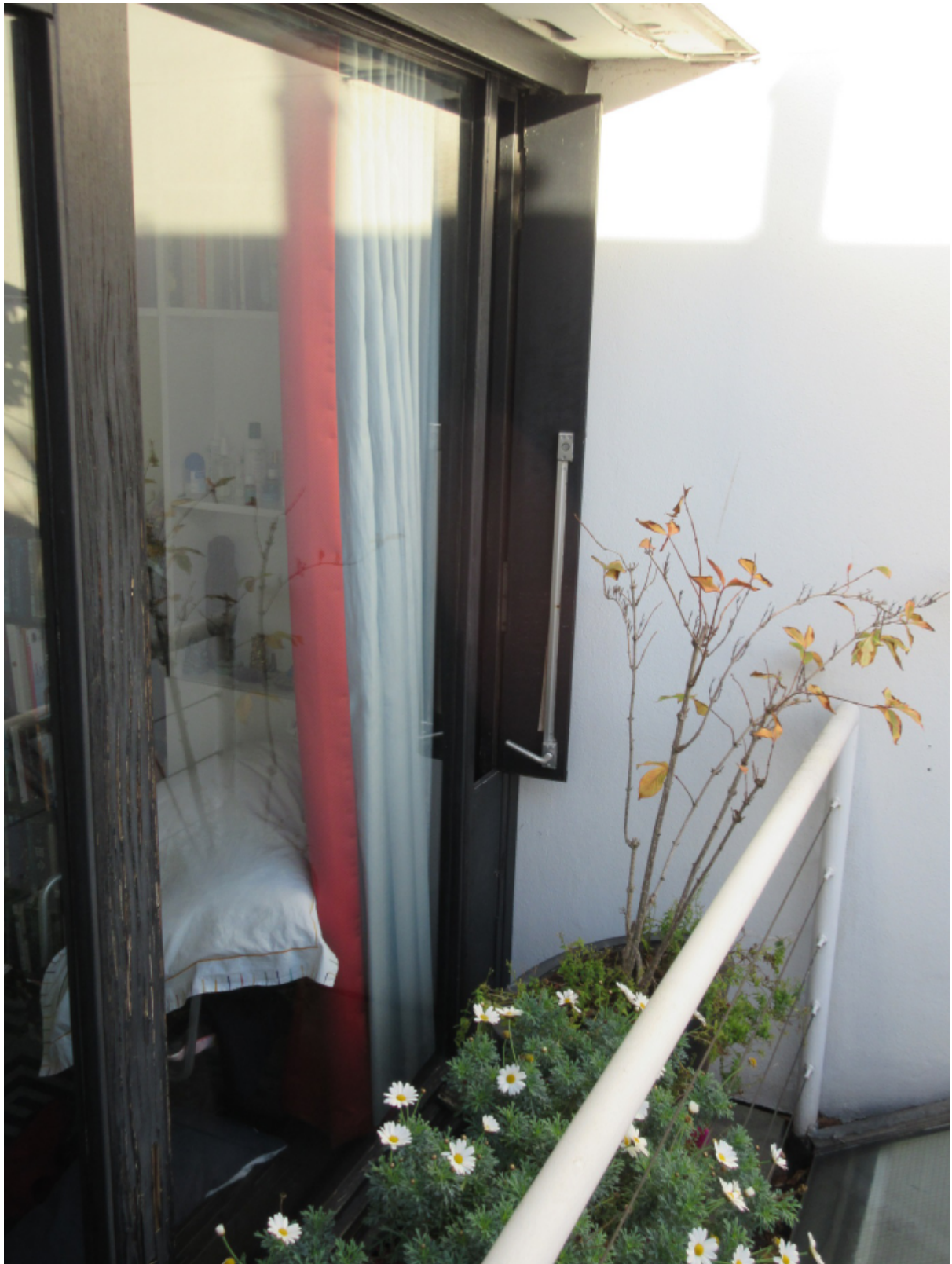
Existing type M rear bedroom sliding doors, consist of a vertical fixed glass panel, two sliding doors and a side vertical panel which can be opened (these vary however across the properties)
