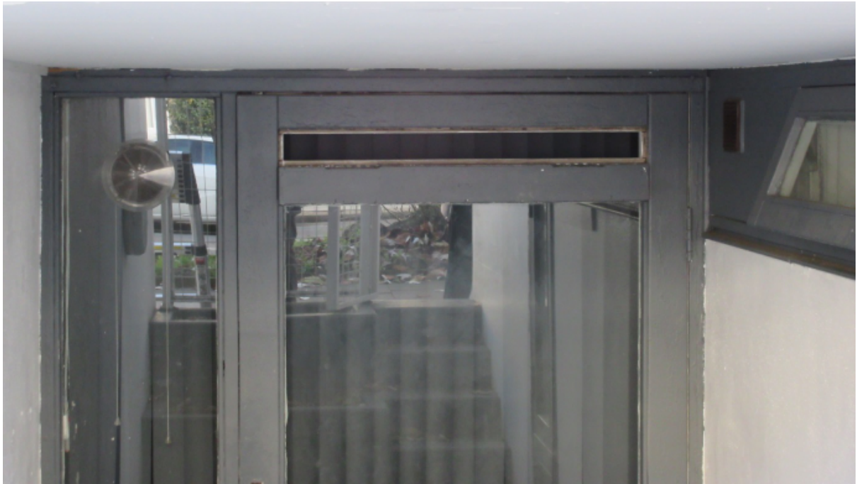
Existing type J front ground floor kitchen facing onto yard, including opening vent panel at the top
