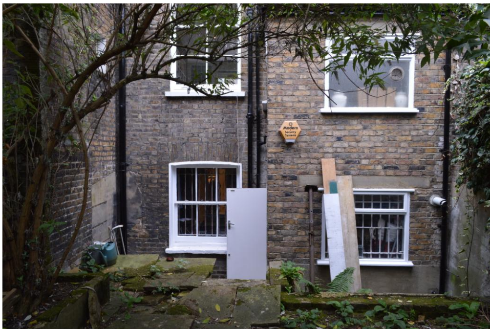
REAR ELEVATION AT BASEMENT SHOWING REAR YARD
