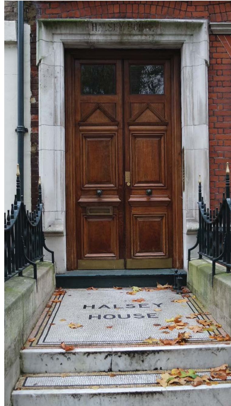
1 ENTRANCE DOORS ON THE SQUARE
