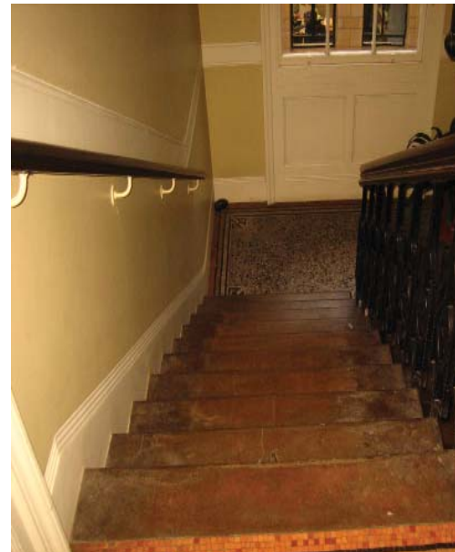
STAIRS AND LANDING
