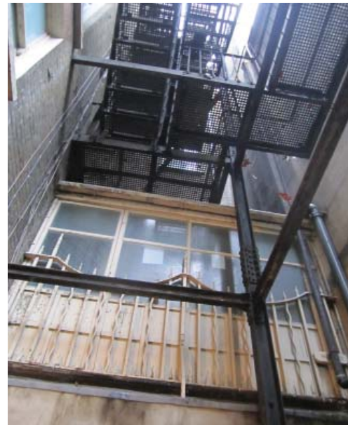
EXTERNAL FIRE ESCAPE
