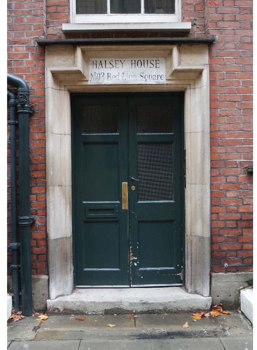
2 ENTRANCE DOORS ON DANE STREET
