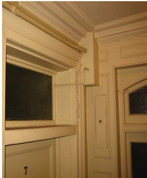
CORNICING TO STAIRWELL
