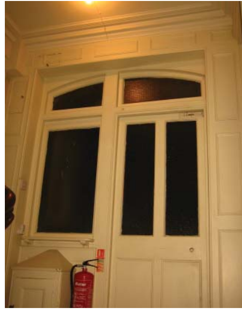
EXISTING LANDING DOORS TO EXTERNAL FIRE ESCAPE
