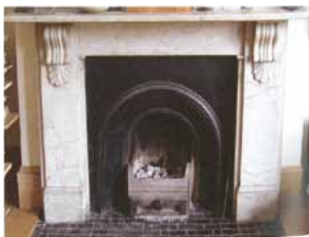
This fire surround has brackets supporting the mantle shelf.
