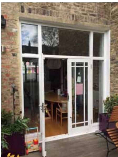
Fig 10. Ground level terrace. Existing double doors onto terrace
