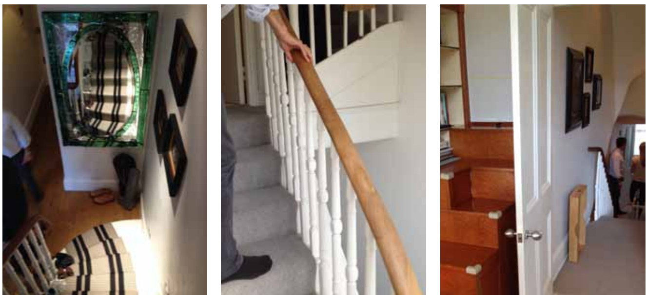
Fig 22. Original staircase photos at ground floor (left), second floor (centre) and stopped up at first floor (right)
