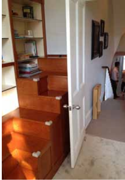
Fig 27. Existing modern joinery over communal staircase to be removed
