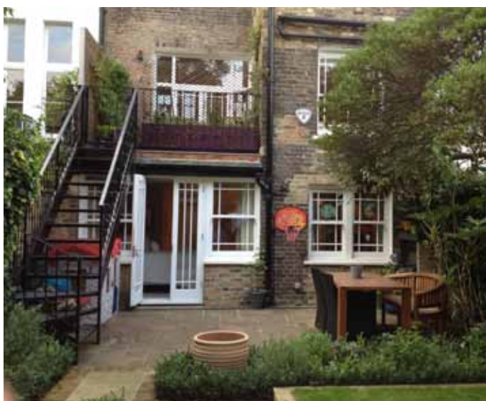
Fig 08. Lower ground level, rear wall. Existing photo
