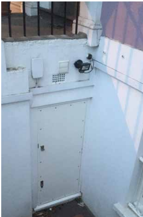
Fig 06. Existing front door to lower ground floor in front light well
