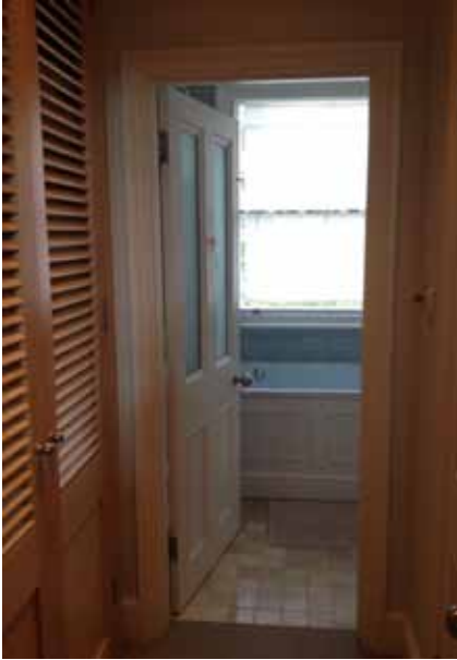
Fig 26. Existing closet wing bathroom to be removed
