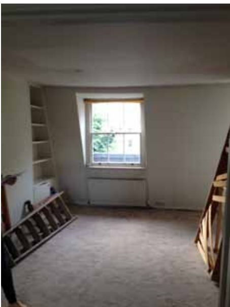
Fig 30. Existing condition of third floor
