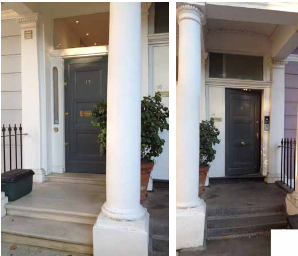
Fig 05. Original main entrance at 17 Chalcot Square (left) and altered entrance at 16 Chalcot Square (right)
