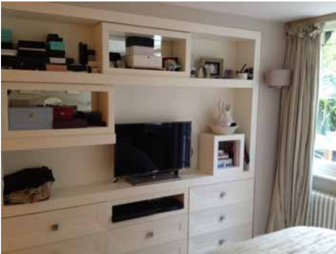
Fig 23. Existing infill joinery to be removed
