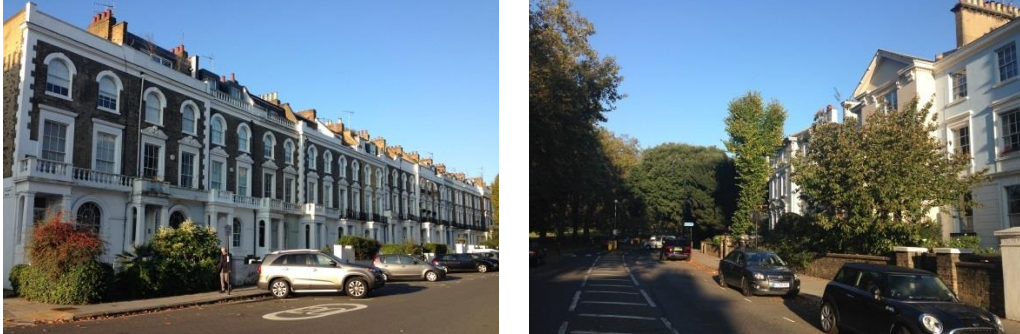
Figure 3.45 – Grand villas and terraced row characterise the conservation area
