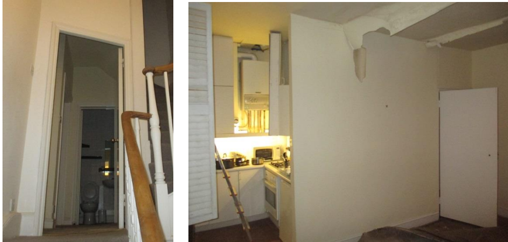
Figure 3.35 – Additional partitions to create a self-contained apartment
