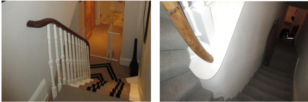
Figure 3.24 – Original staircase blocked between first and second floor, though the bannister may have been retained within the wall
