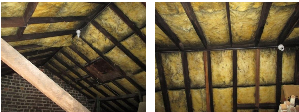
Figure 3.15 – Historic roof structure supplemented in places with modern beams
