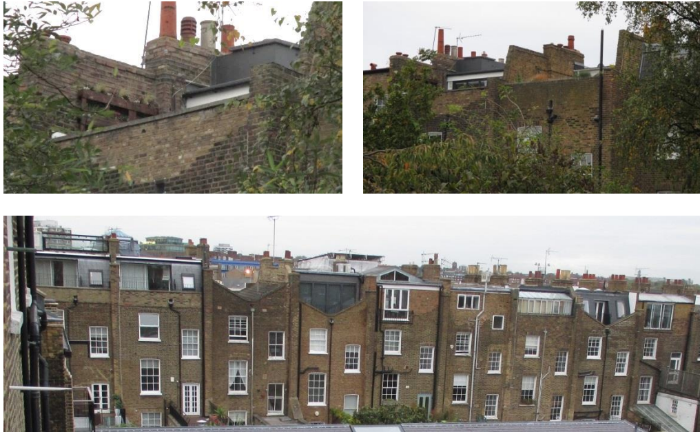
Figure 3.9 – Varied roofscape in the surrounding conservation area
