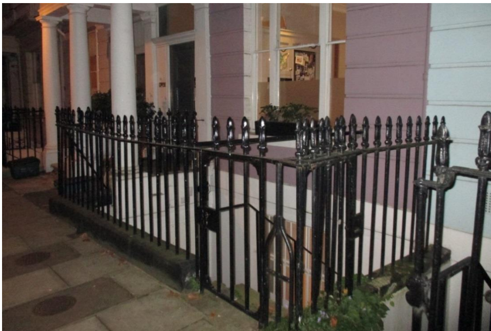
Figure 3.11 – Front boundary railings
