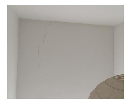
Minor crack in wall above staircase at second floor level
