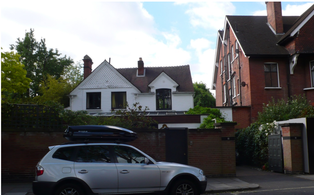
Photo 1 – Street elevation of 10 Nutley Terrace.
