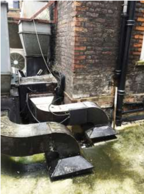
Existing duct and fresh air intake on the existing rear roof
