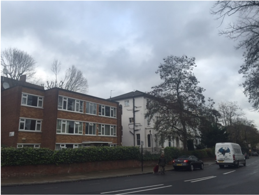
Photo 2: View towards no.150 from Quex Road (looking north east).
