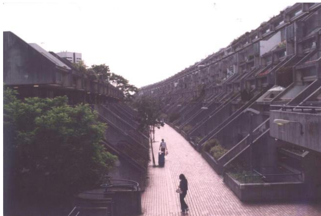
Rowley Way: As existing – painted balconies
