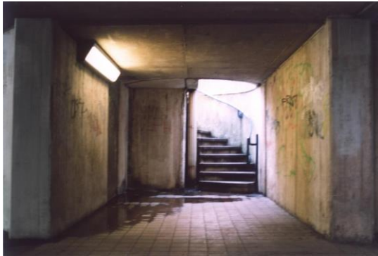
Existing: Poor quality service areas.
