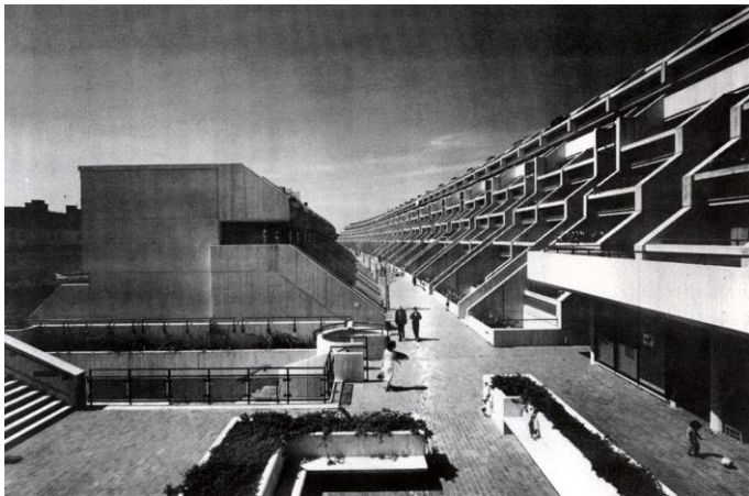
View looking West along Rowley Way
