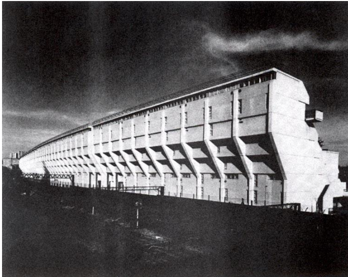
Rear Elevation Facing Train Line to the North
