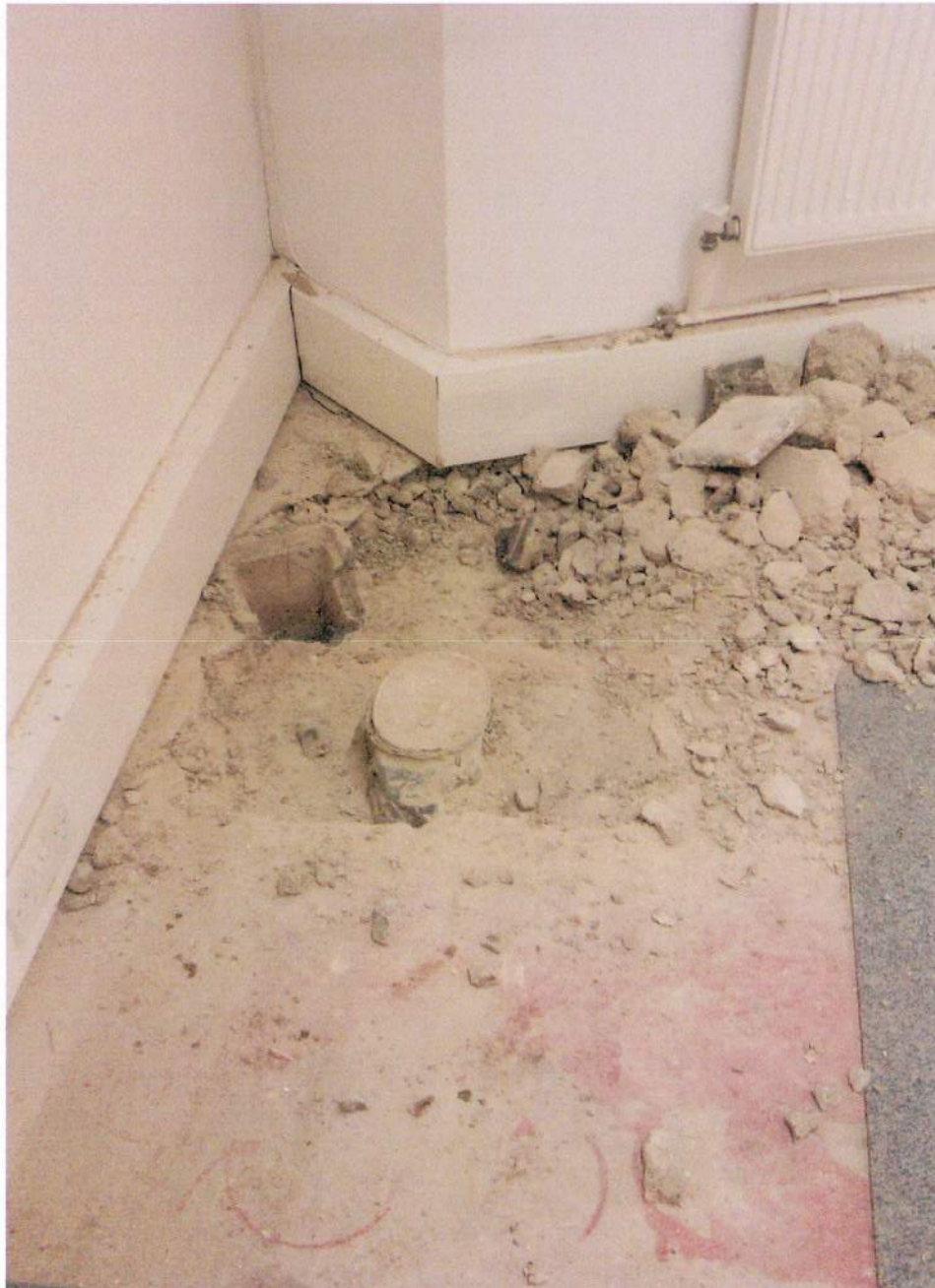
View of the findings encountered in Trial Pit No 8, looking south
