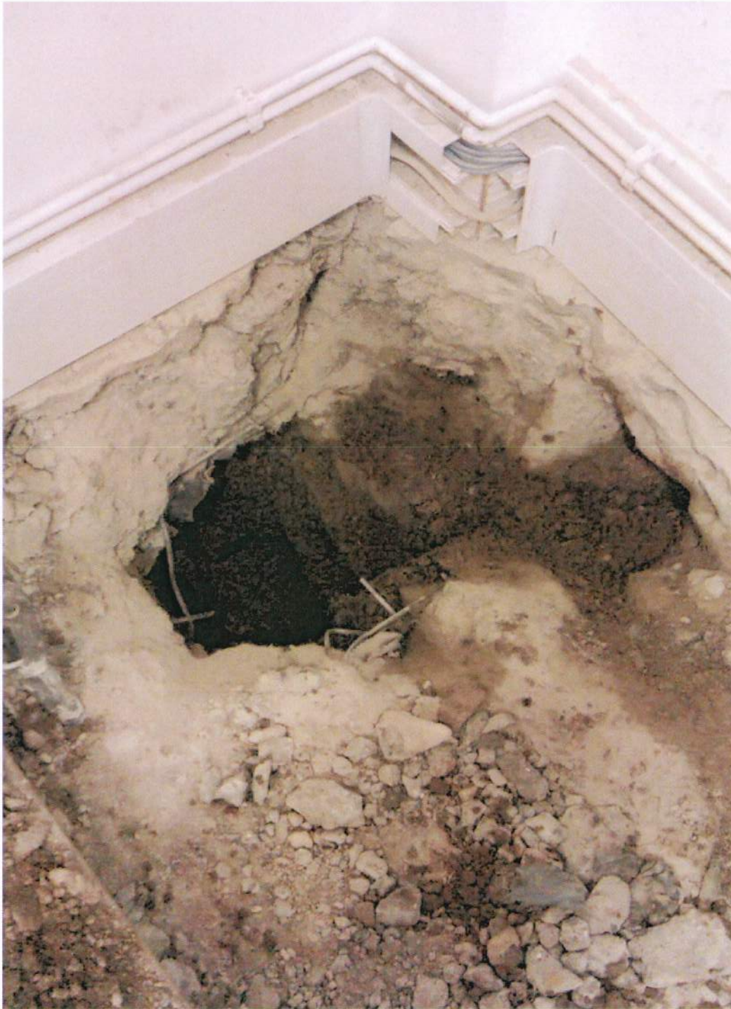
View of the findings encountered in Trial Pit No 7, looking southeast
