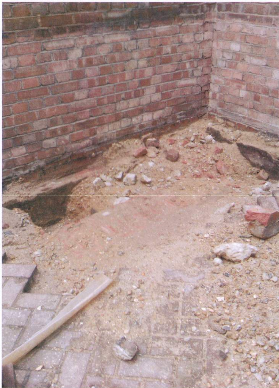
View of the findings encountered in Trial Pit No 5, looking northwest
