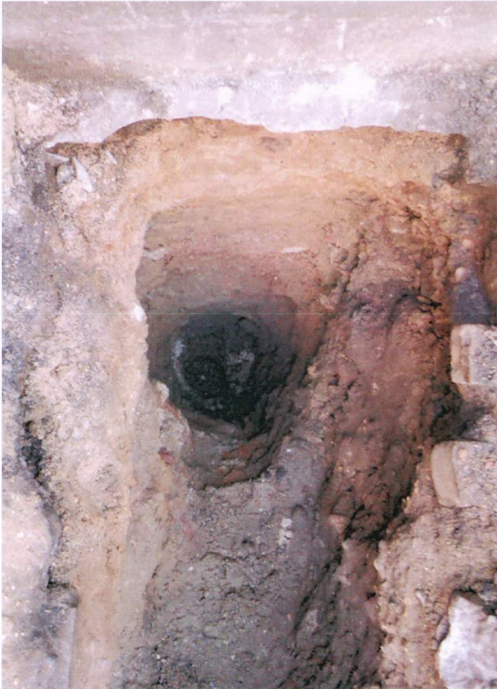
View of the footings encountered in Trial Pit No 3, looking south
