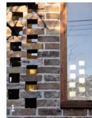
1 Open-jointed brickwork
