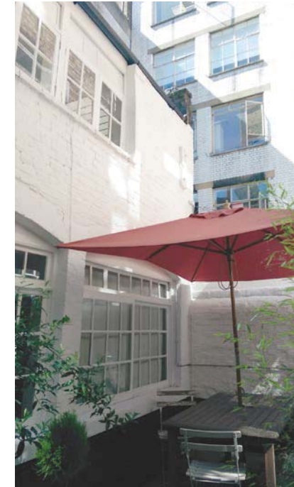
Mews building to no. 6 Denmark St
