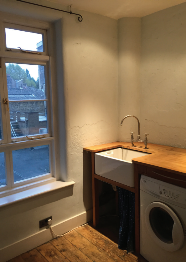
FIG 4: EXISTING FIXTURES ADJACENT TO PROPOSED OPENING (LHS)
