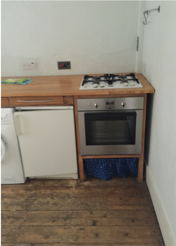
FIG 5: EXISTING FIXTURES ADJACENT TO PROPOSED OPENING (LHS)
