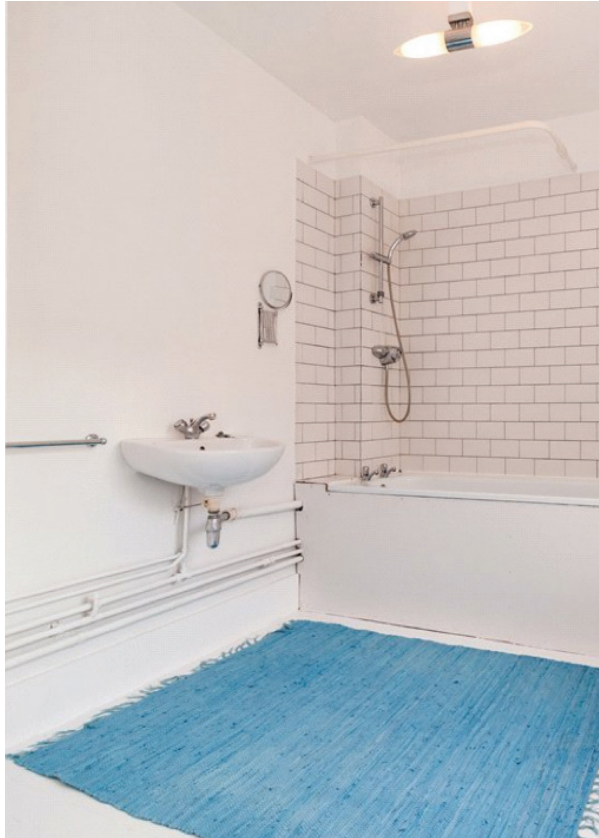
FIG 3: EXISTING FIXTURES ADJACENT TO PROPOSED OPENING (RHS)
