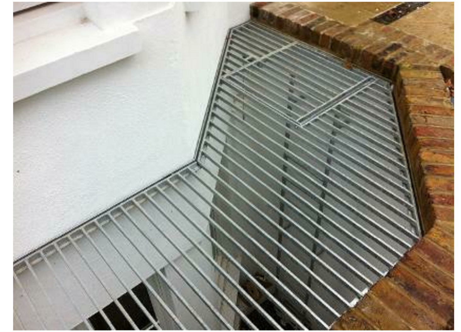
Sample Photo to show basement grill
