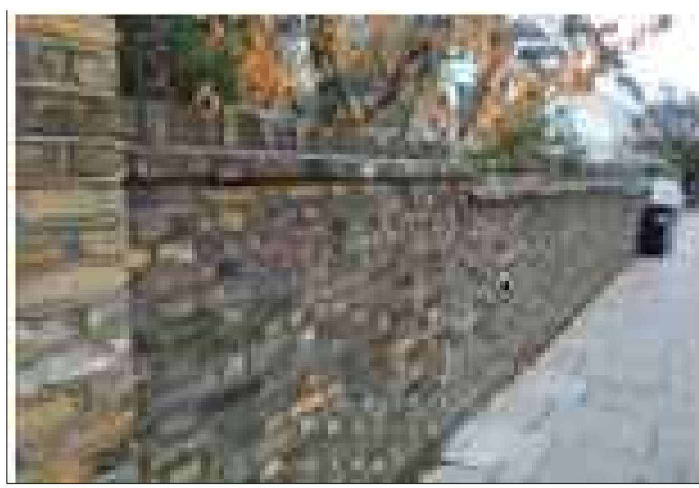
Rebuilt Garden Wall
