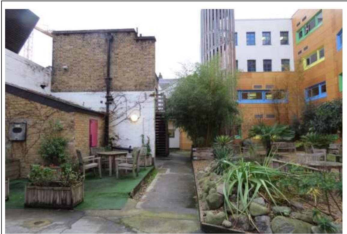
Photograph 9 (TN8): Courtyard to the south of the building
