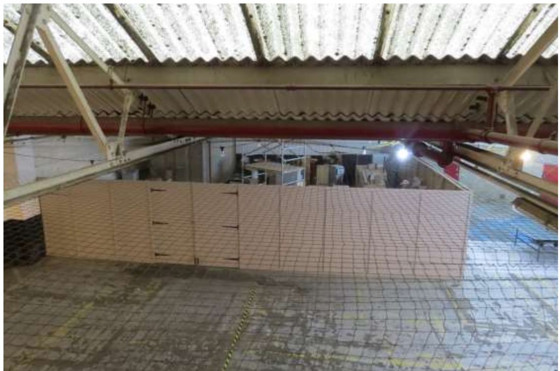
Photograph 8 (TN7): North-western storage area. Bird netting covering the full extent of the roof
