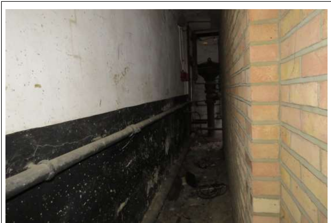
Photograph 5 (TN4): Cavity space behind the north-eastern substation
