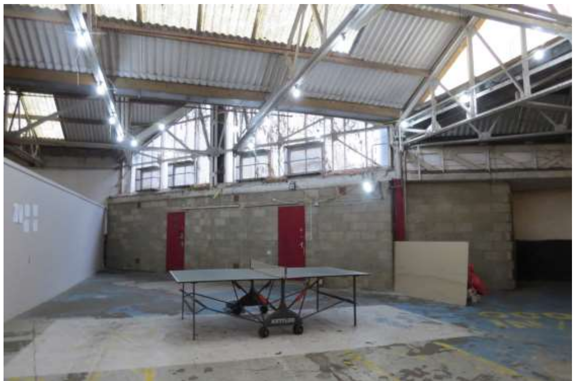
Photograph 6 (TN5): Northern storage rooms
