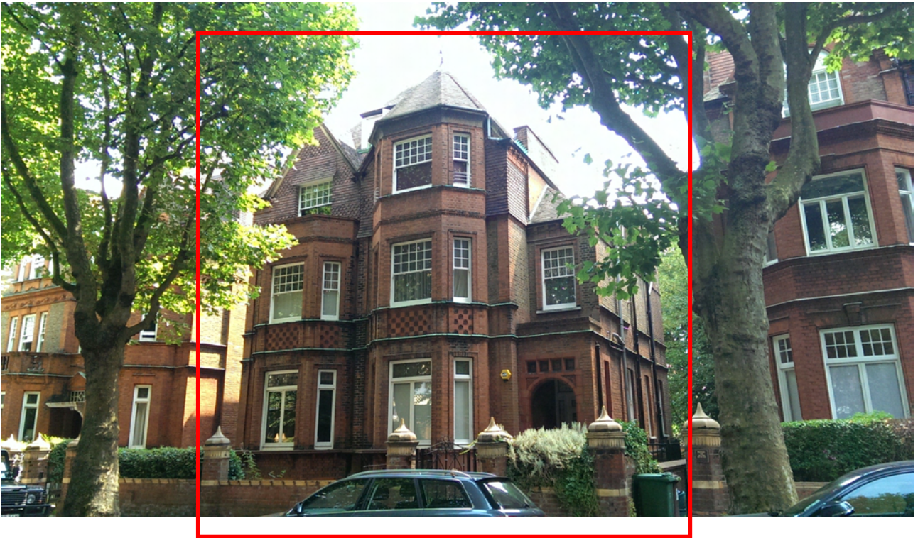
Photograph 1 showing the front (main) existing elevation:
