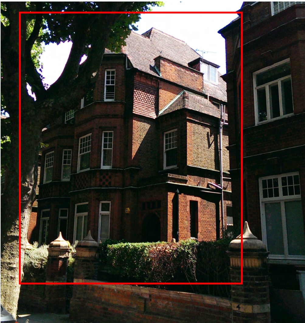
Photograph 2 showing the existing side elevation (please note existing dormer window):
